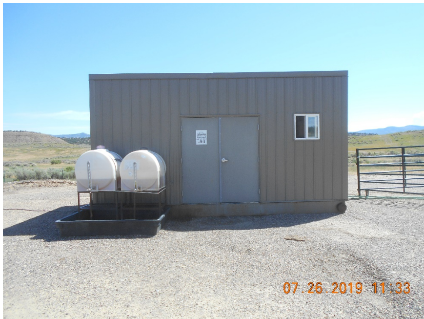
Pump housing. Chemical drums with secondary containment.
