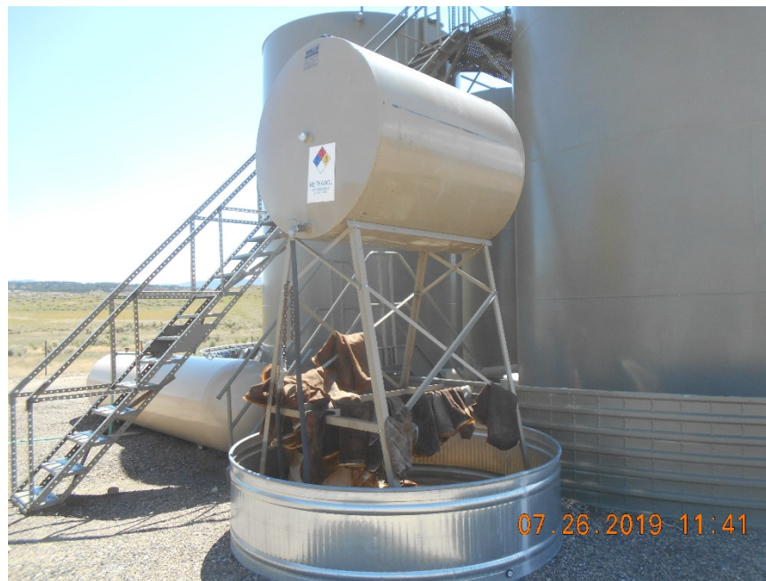
Methanol tank with secondary containment.
