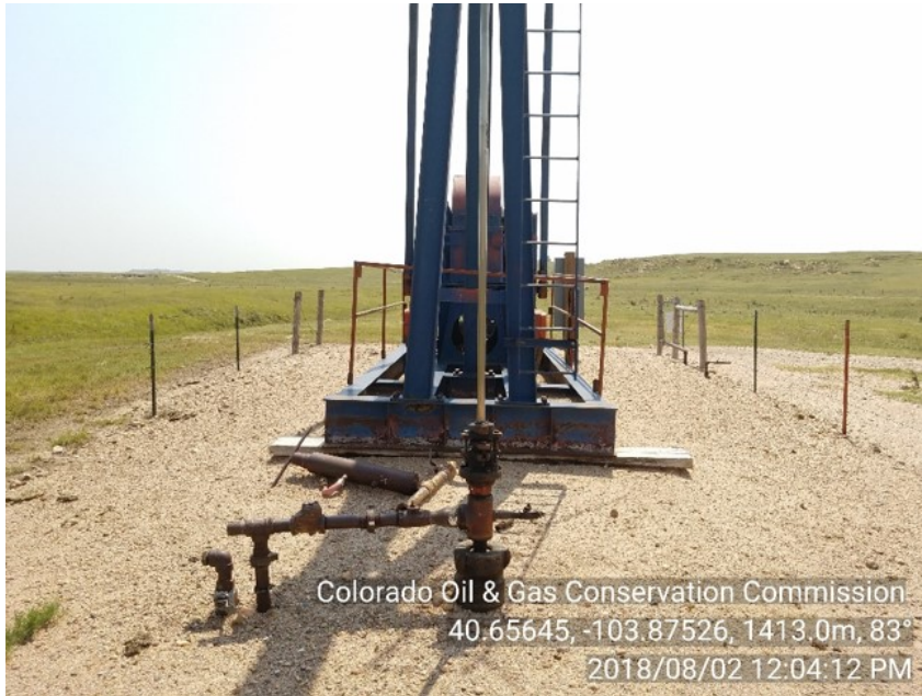
Photo #1 Sooner Unit 13-16 (05-123-13452) Wellsite Bradenhead NOT plumbed to surface Unused Equipment previous insp.
