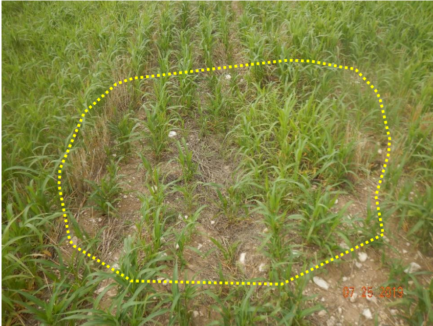
Photo 1: Photo taken from the well. Subsidence remains evident at the well location.
