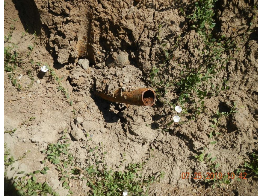
Close up of steel pipe in sidewall of excavation.
