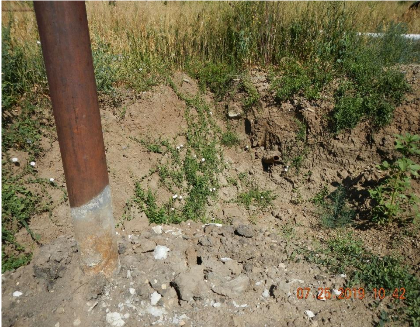
PA marker with 2" steel pipe protruding from sidewall of excavation.
