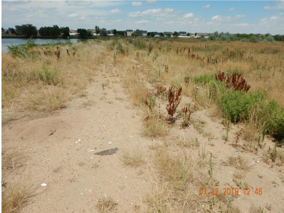
Photo 1. Photo taken from a portion of the access road, facing North. Operator has failed to perform final reclamation activities throughout the access road. Photo illustrates the access road with gravel and no evidence that final reclamation activities occurred. In addition, noxious weeds (Musk and Scotch thistle) were observed throughout portions of the access road and well location.
