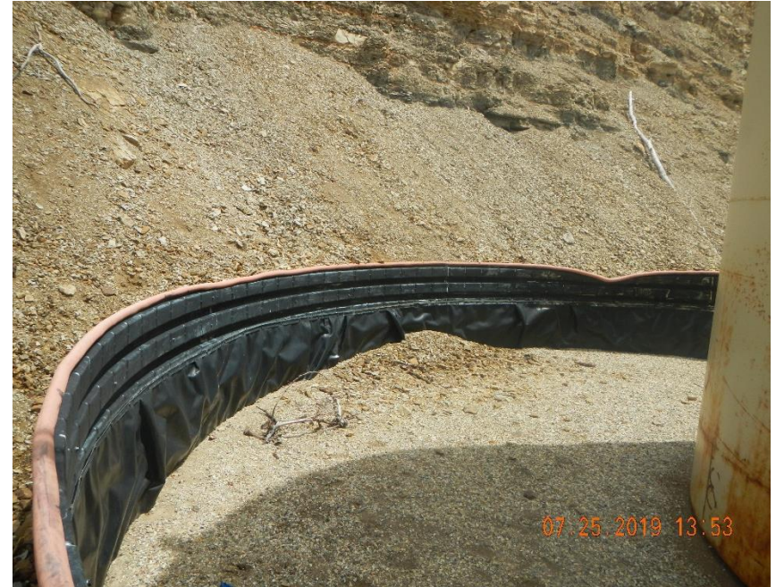
Sediment and shale inside tank berm..
