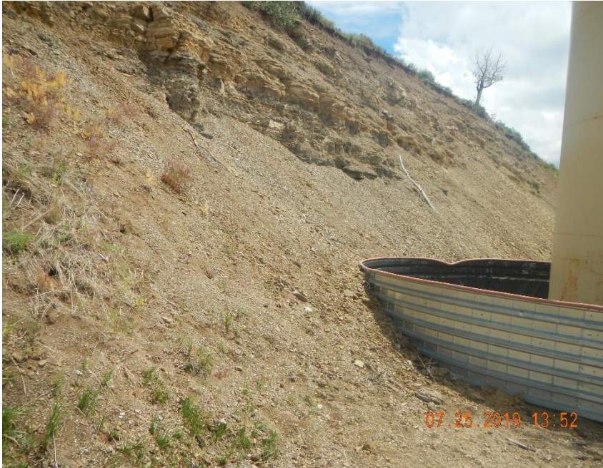
Sediment and shale sloughing off of cut slope .
