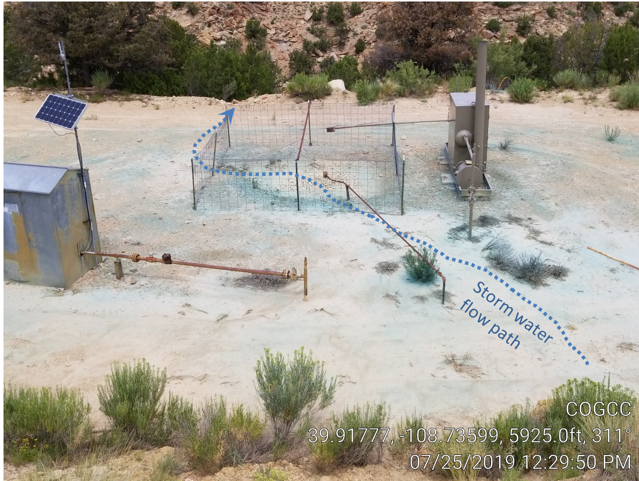
Photo 2. Meter building, pit, and separator.
