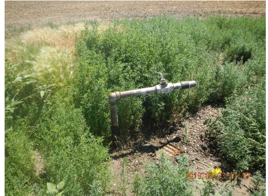
Photo 8: Furthest E flow line riser on E side of production facility.
