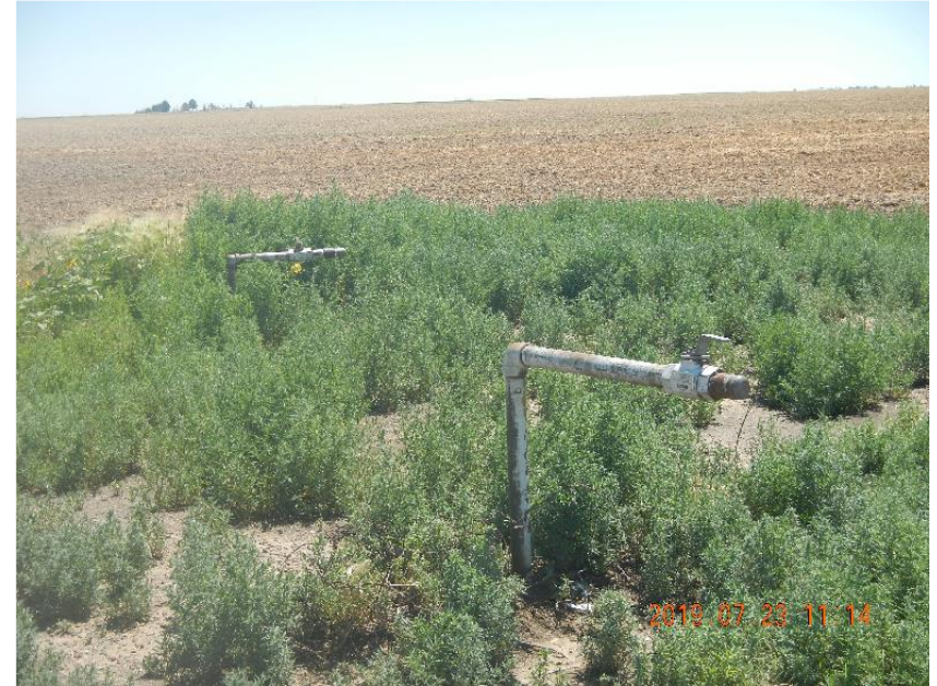
Photo 10: View of both flow line risers on production facility.
