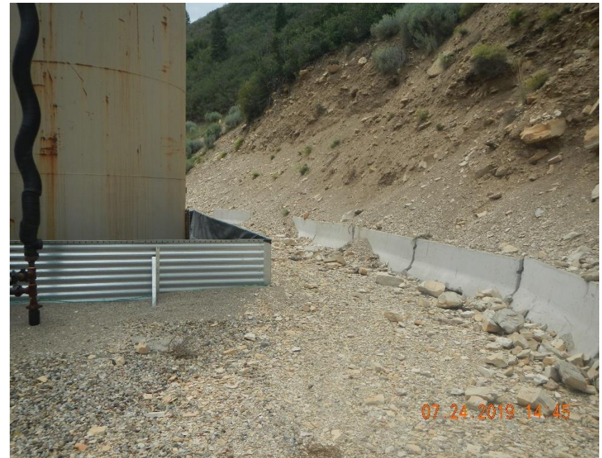
Cut slope behind tank battery is sloughing sediment over bmps.
