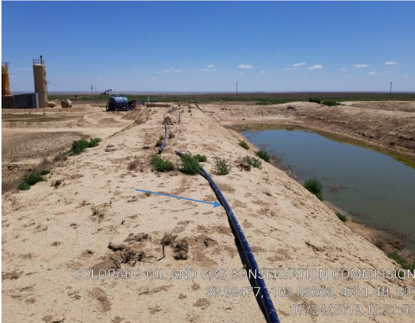
Pic 13 fiberglass tubing on pit berm
