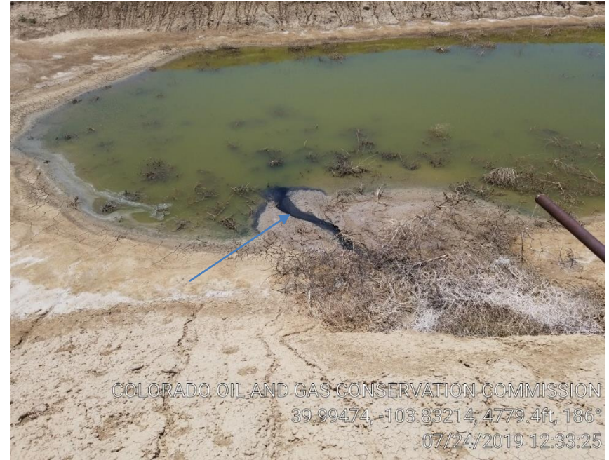
Pic 17 Possible hydrocarbons in pit/no netting
