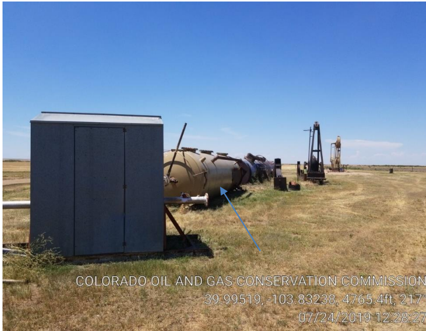
Pic 3 storage of equipment
