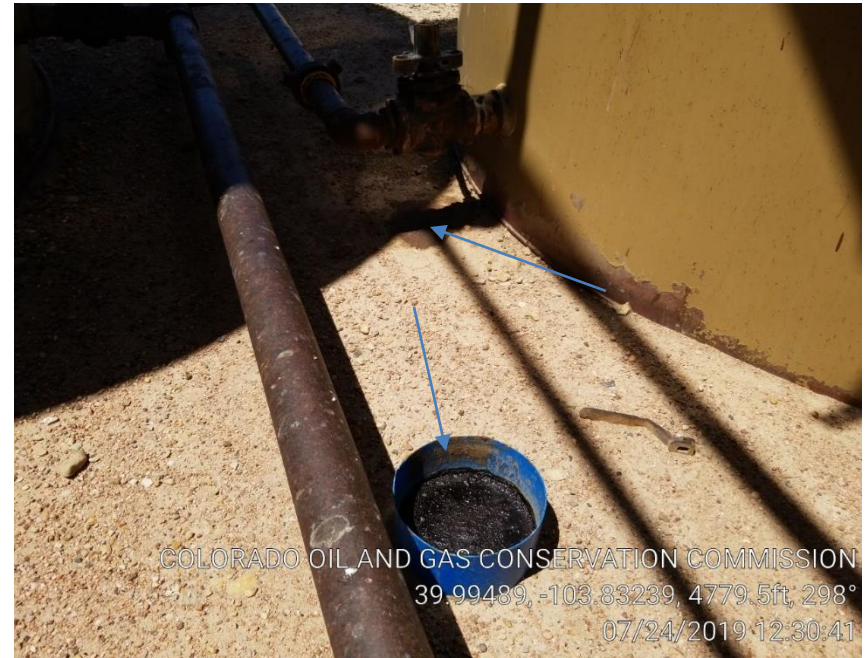
Pic 10 stained soil below valves/bucket with unknown substance
