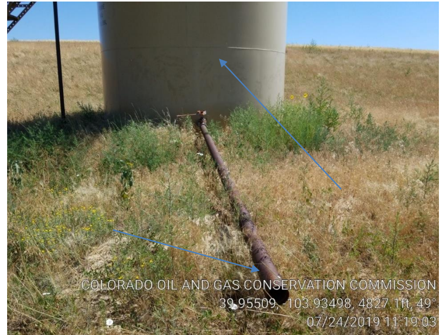
Pic 10 tank no sign, placard, berm in disrepair, no cap on line
