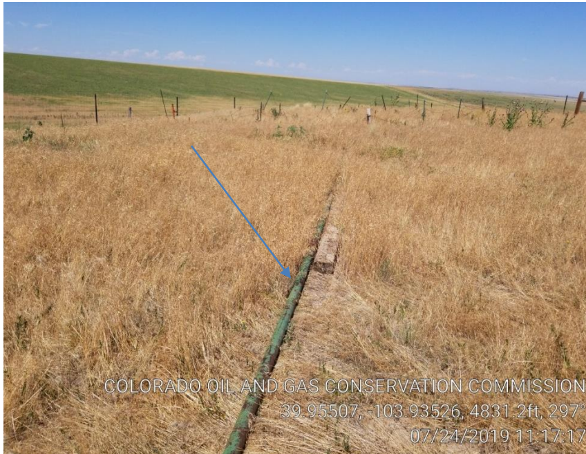
Pic 7 unused 2" line going to pit
