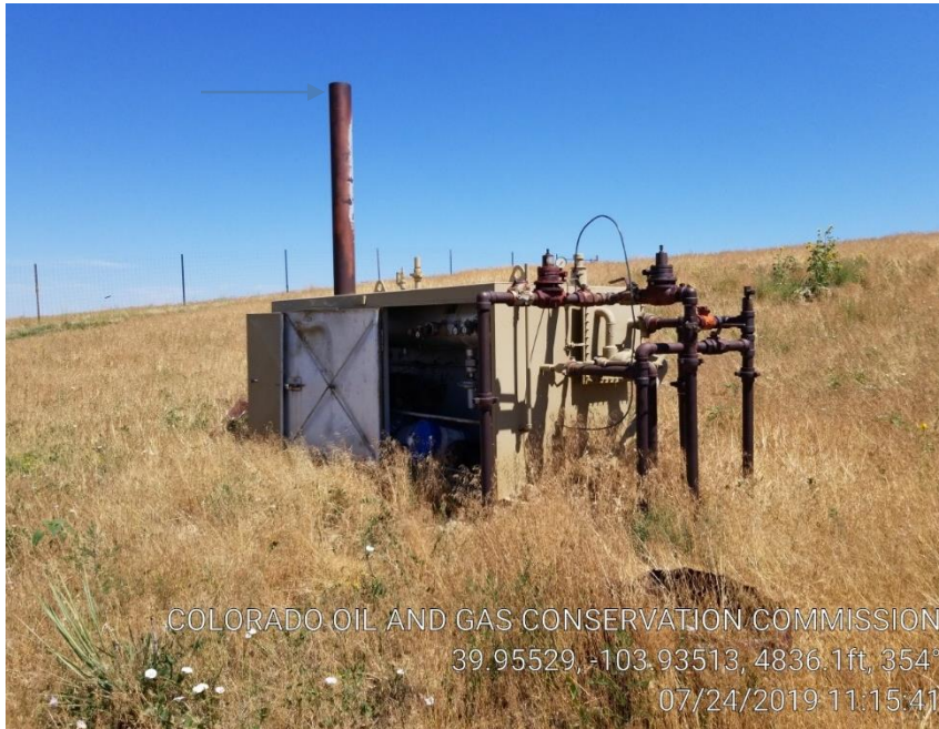
Pic 3 separator with no bird protector
