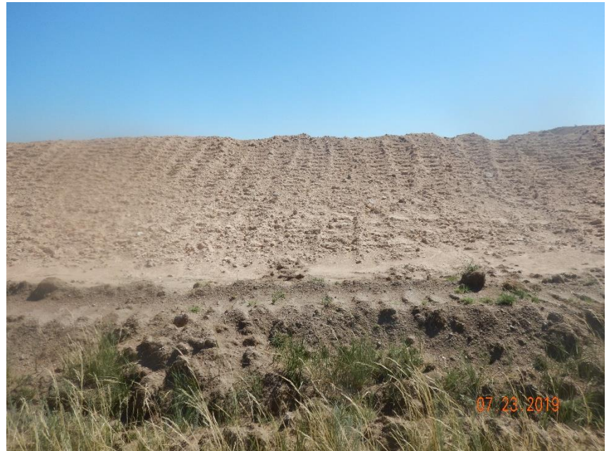
Photo 6: Photo taken from the west end of the location, facing east. Photo shows tracking on slopes appear to be in proper functioning condition.
