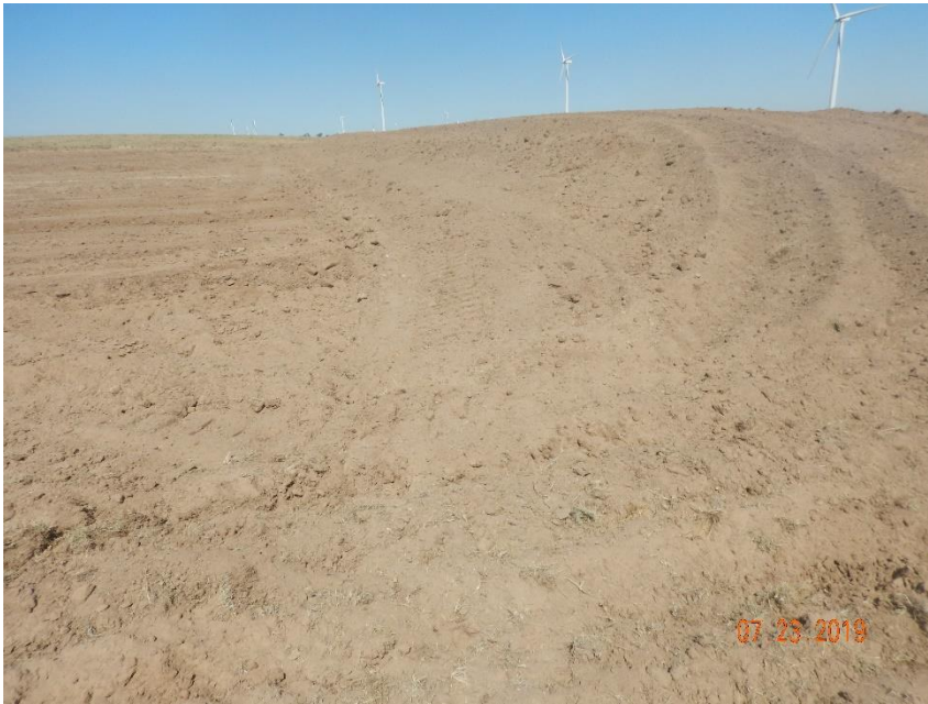
Photo 5: Photo taken from the north end of the location, facing northwest. Photo shows topsoil stockpile. Soil salvage in process at time of inspection. Stabilization BMPs will need to be installed to protect from stormwater/wind have not been installed in accordance with 1002.c
