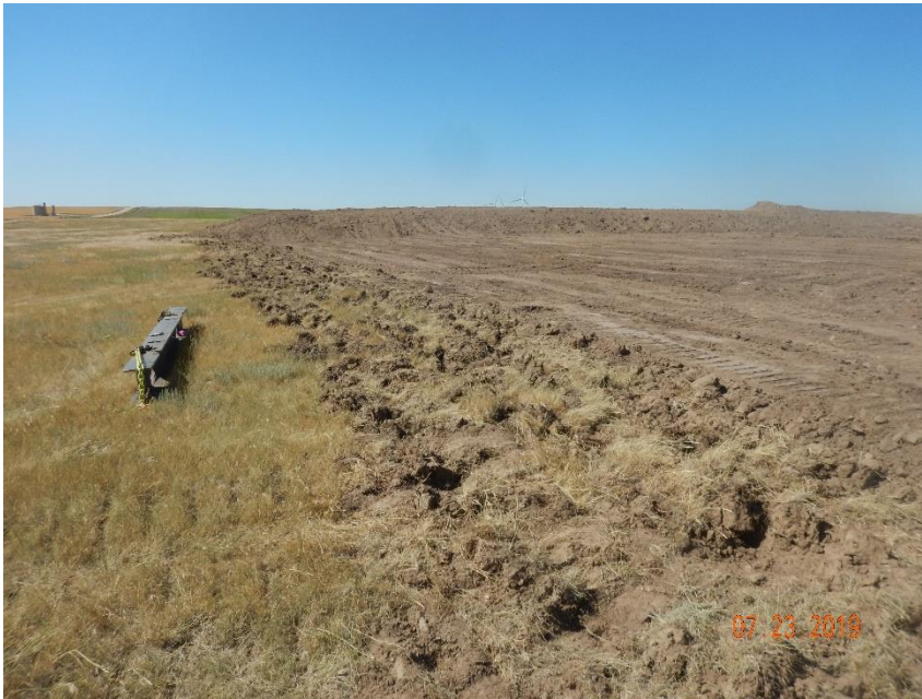
Photo 1: Photos 1-4 taken from the east end of the location, facing south, southwest, northwest to north. Photos show construction in process. Photos also show surface roughening stormwater BMP has been installed along perimeter of the location/disturbance.
