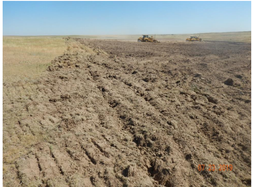
Photo 6: Photo taken from the southwest corner of the location, facing north. Photo shows construction in process. Photo also show surface roughening stormwater BMP has been installed along perimeter of the location/disturbance.
