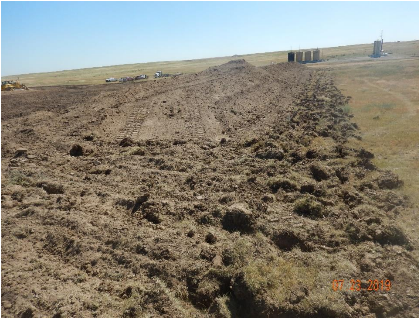
Photo 7: Photo taken from the southwest corner of the location, facing east. Photo shows construction in process. Photo also show surface roughening stormwater BMP has been installed along perimeter of the location/disturbance.
