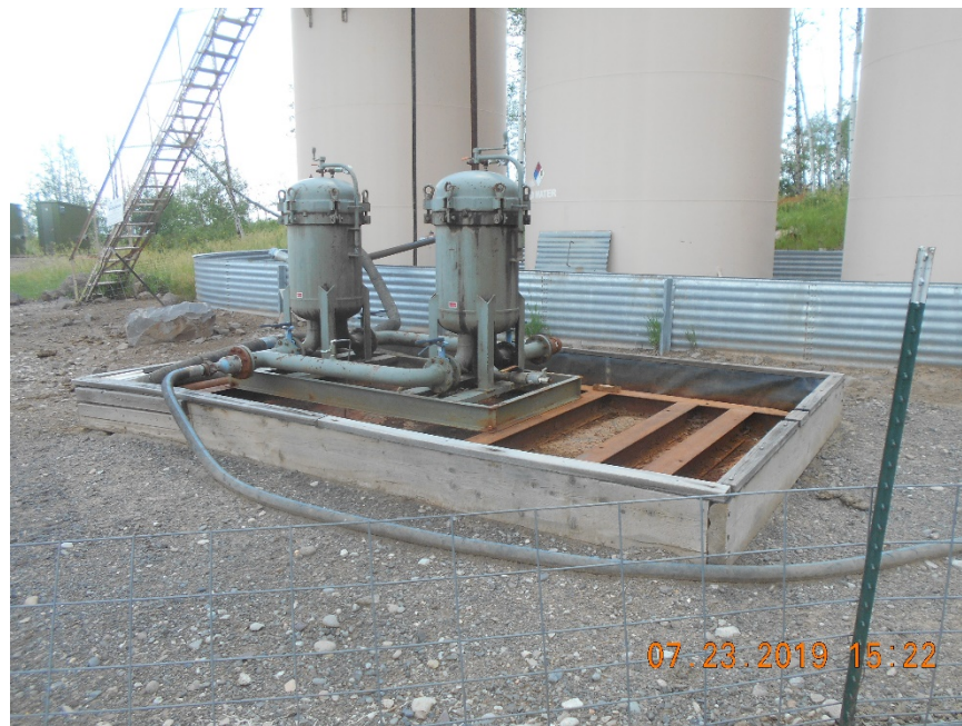
Filter housings inside secondary containment.
