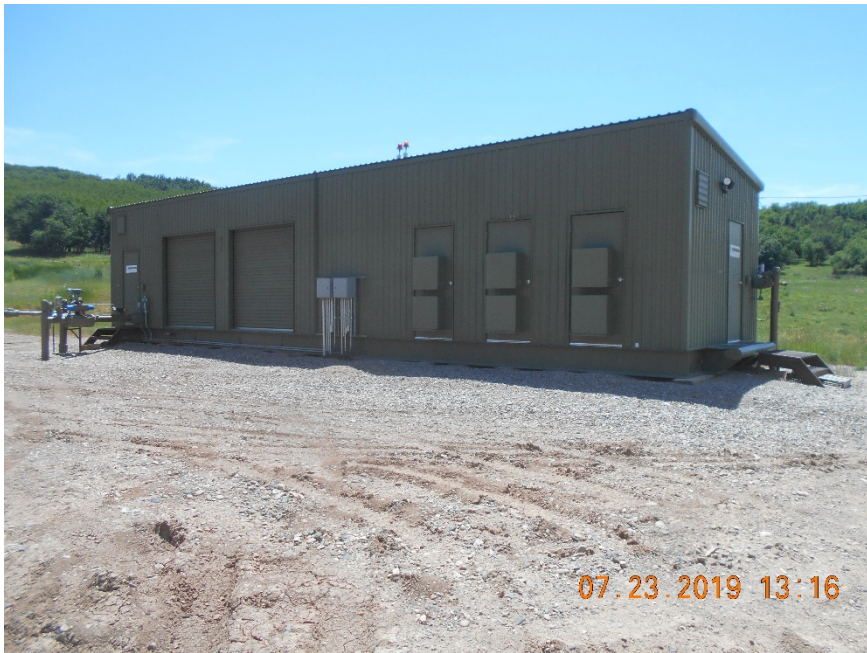
Pump and Generator Housing
