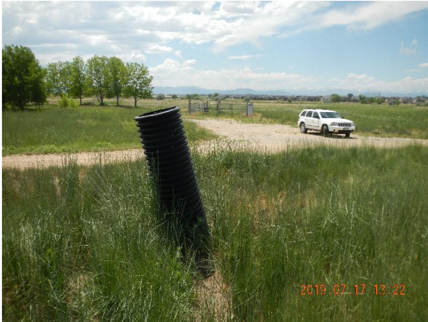
Photo 5: Black plastic culvert over T-Post marking riser location.
