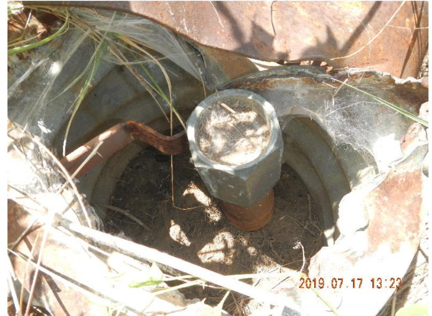
Photo 8: Close up view of 2" steel line with open ended valve.
