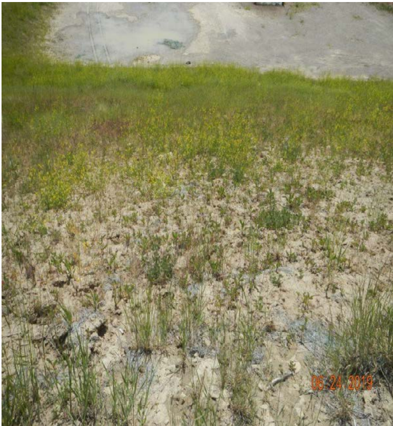
Photo#12: Cut slope has spotty establishment of desirable vegetation.
