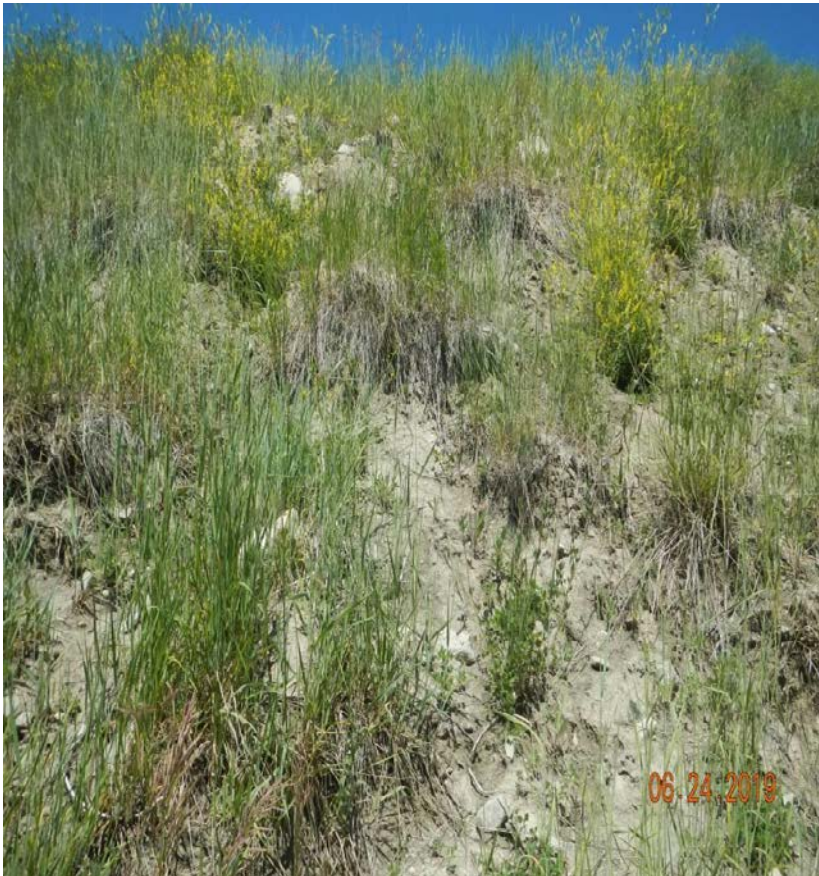
Photo#10: Fill slope has areas of spotty establishment of desirable vegetation.
