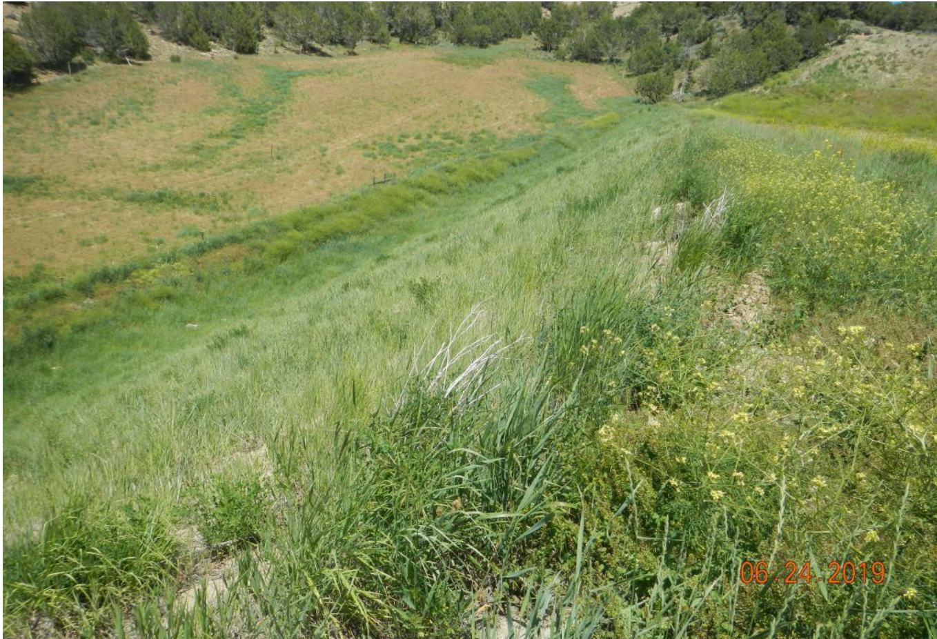
Photo#14: North fill slope has good establishment of desirable vegetation.
