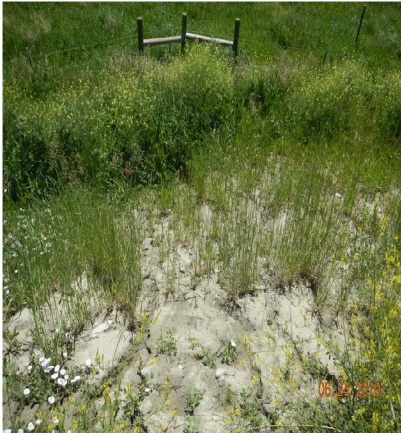
Photo#8: Fill slope has areas of spotty establishment of desirable vegetation.
