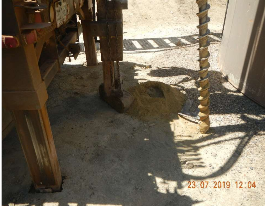
Photo #5 – View of one of the boreholes.
