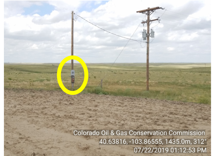
Photo #4 Sooner Unit 2-28 UIC Wellsite Plugged & Abandoned | PA Most unused equipment removed. Unused Electrical panel & pole needs removed.
