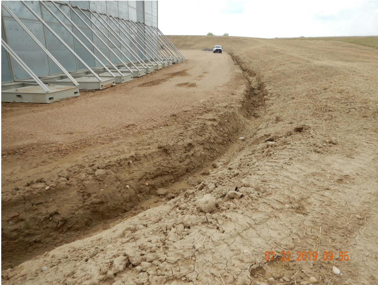
Photo 5. Photo taken from the northwestern well pad, facing South. Photo illustrates a ditch BMP that is directed to a stabilized outlet. It appears the Operator is in-process of installing rip-rap along the ditch BMP.
