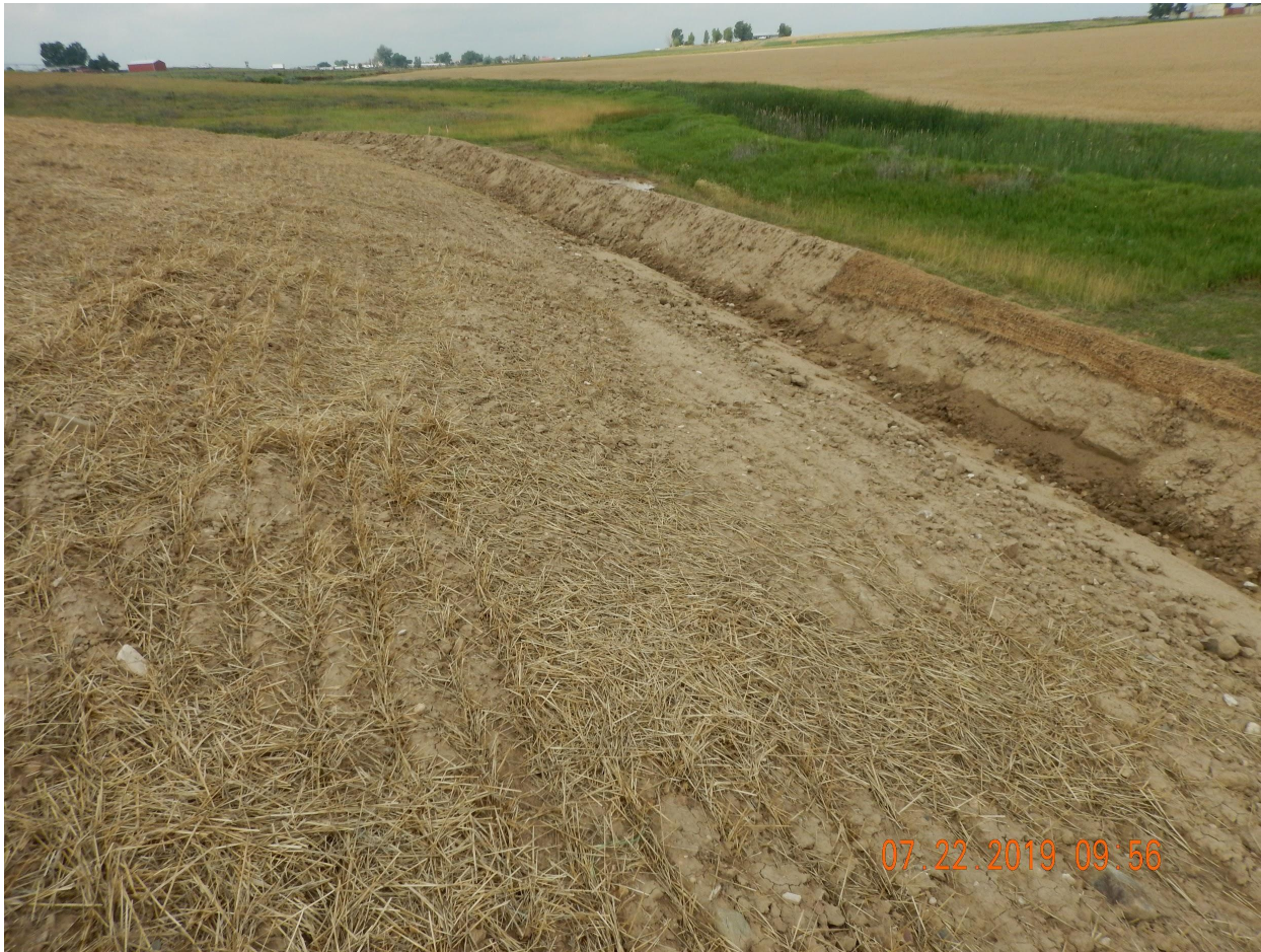
Photo 7. Photo taken from the northwestern perimeter of location, facing West. Photo illustrates a ditch and berm BMP that has been installed in conjunction with a stabilized outlet. Portions of the berm BMP have been stabilized with erosion control blankets.
