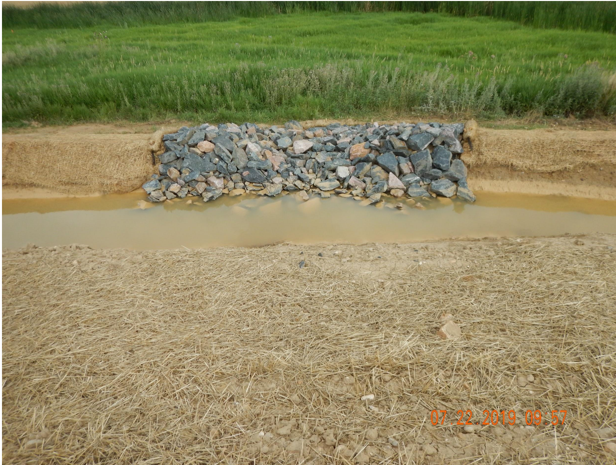
Photo 9. Photo taken from the northeastern perimeter of location, facing North. Photo illustrates a stabilized outlet.
