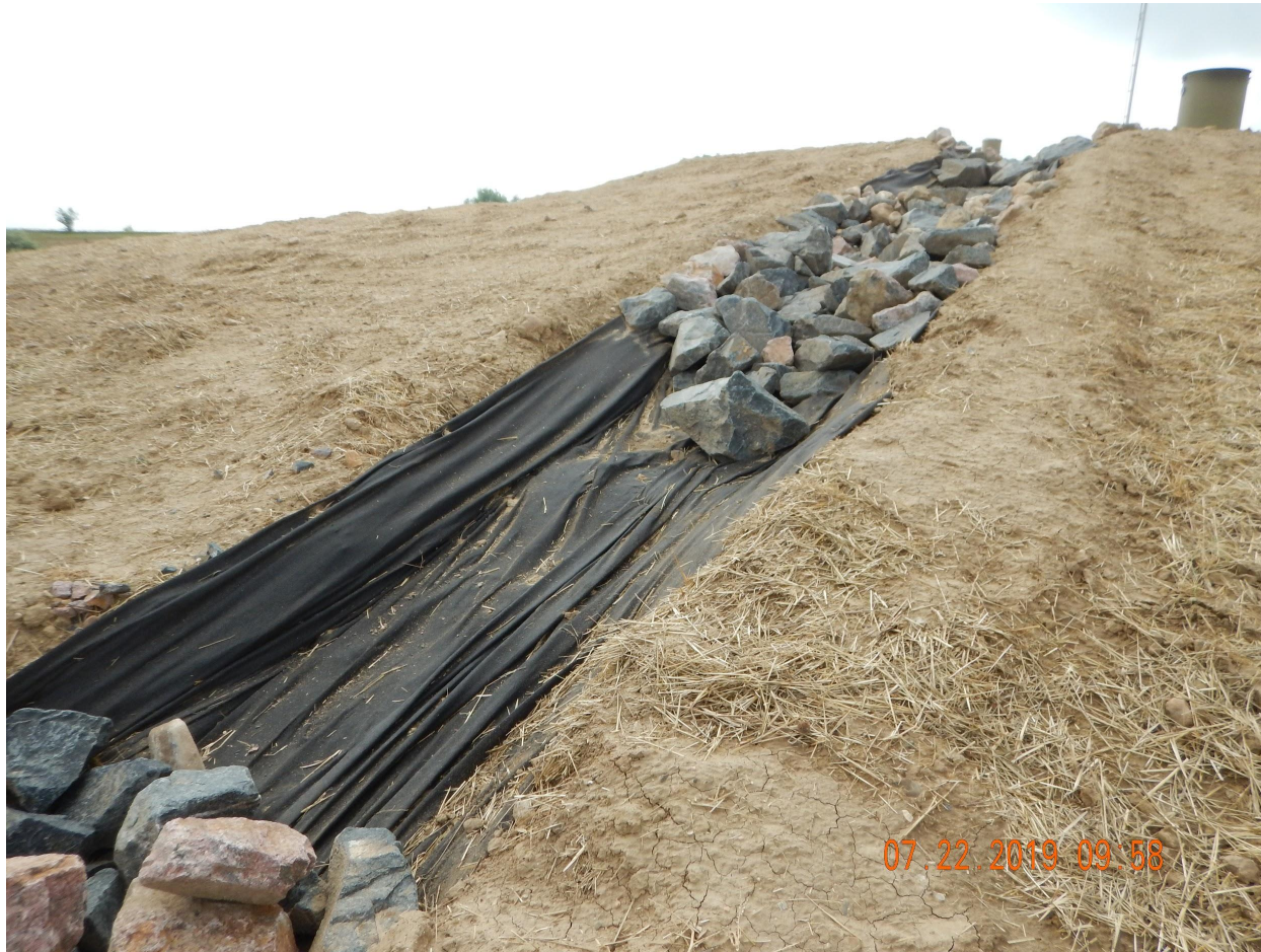
Photo 11. Photo taken from the northeastern perimeter of location, facing South. Photo illustrates a stabilized channel (in-process) that is directed to a stabilized outlet.
