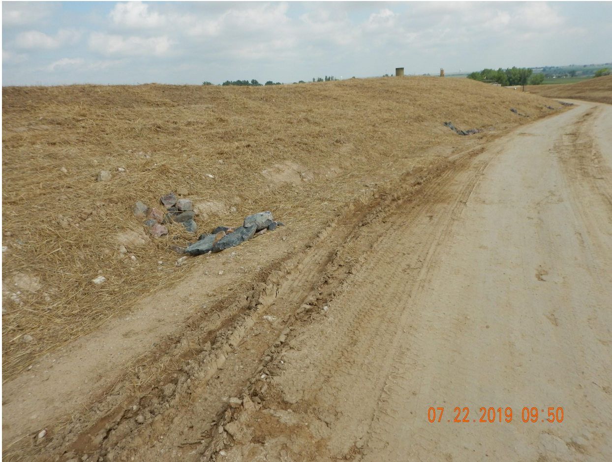
Photo 1. Photo taken along a portion of the access road, facing North. Photo illustrates the Operator has seeded and straw crimped mulch throughout the interim areas. Also, Operator has installed rip-rap as check dams along the access road ditch. BMP maintenance is required along a section where truck traffic damaged the BMPs.
