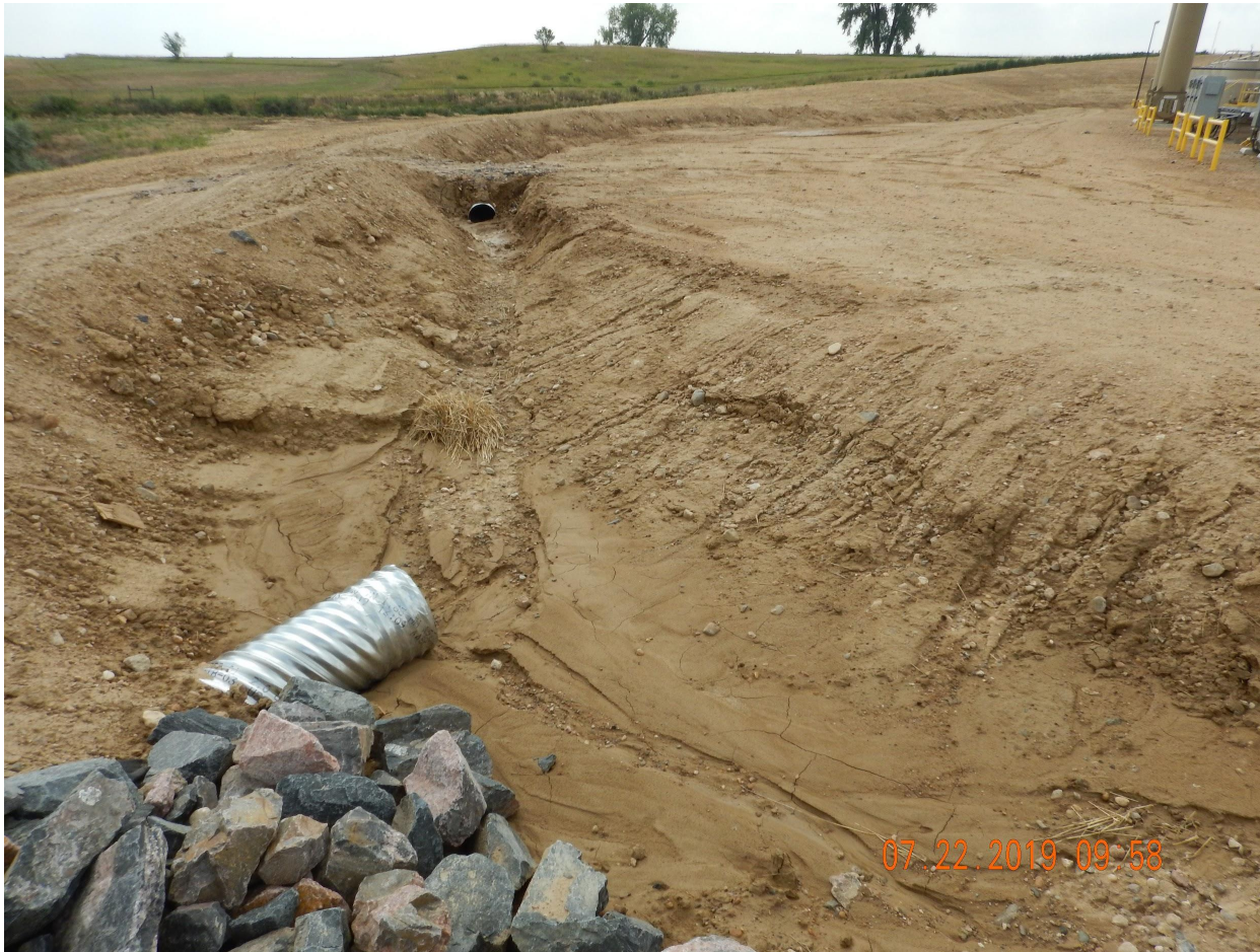
Photo 12. Photo taken from the northeastern well pad, facing East. Photo illustrates an inlet area that is in-process of being stabilized with rip-rap.
