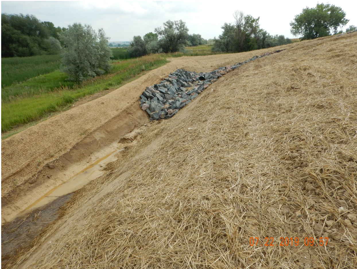
Photo 10. Photo taken from the northeastern perimeter of location, facing East. Photo illustrates a stabilized outlet area of the culvert.
