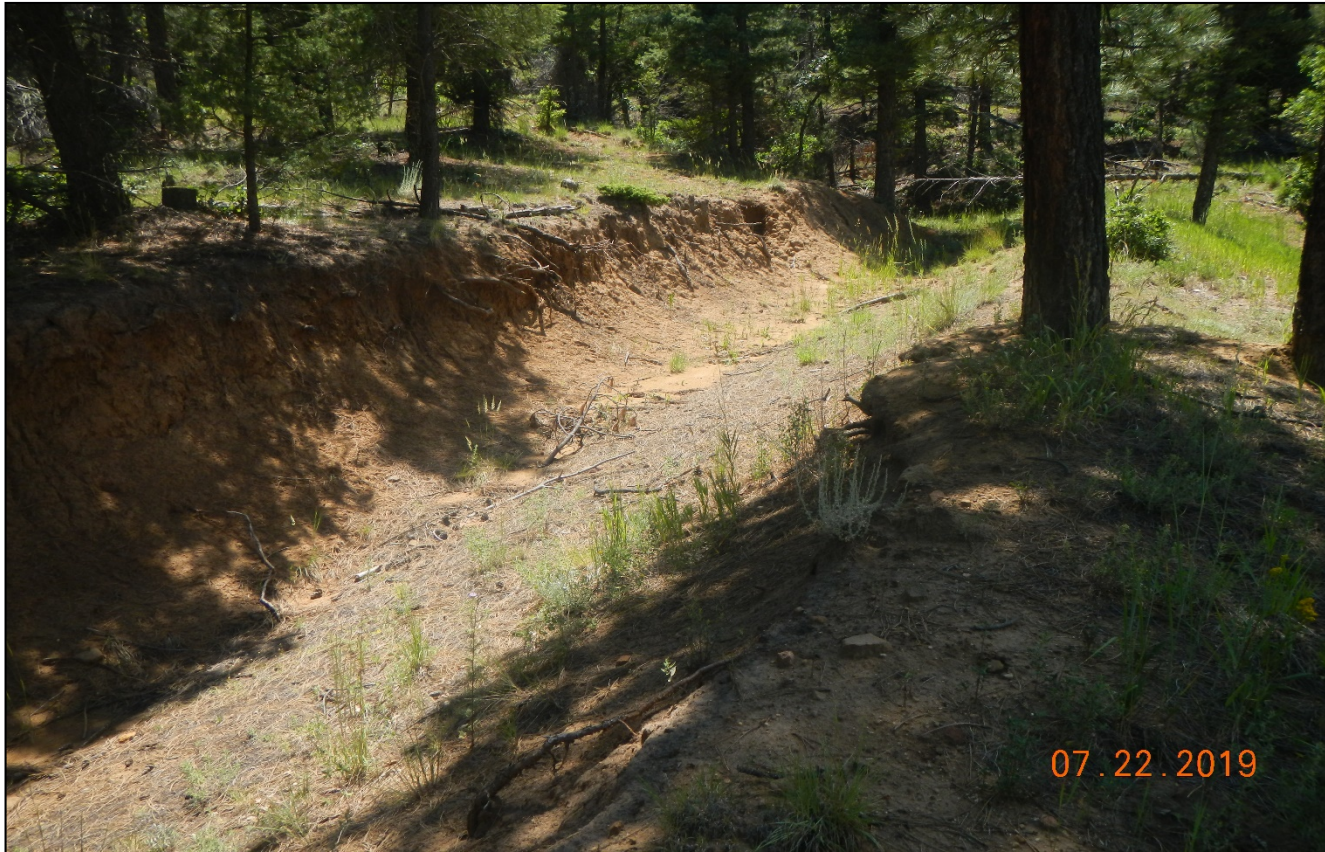
Photo 6. There is a perimeter ditch that diverts drainage around the location.
