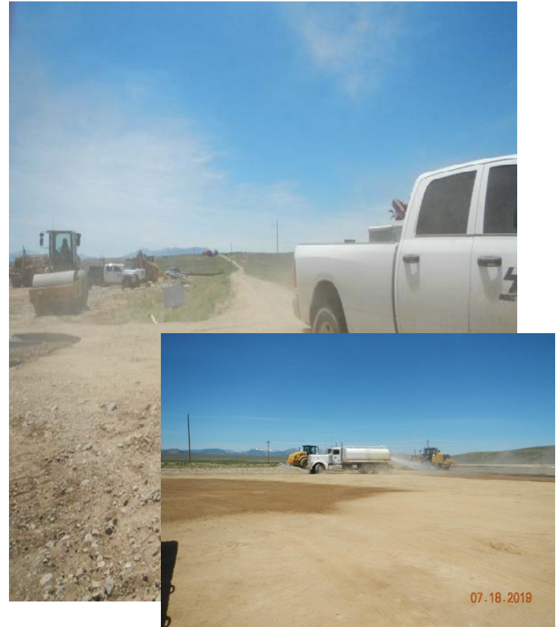
Photo#10: Fugitive Dust; water truck working
