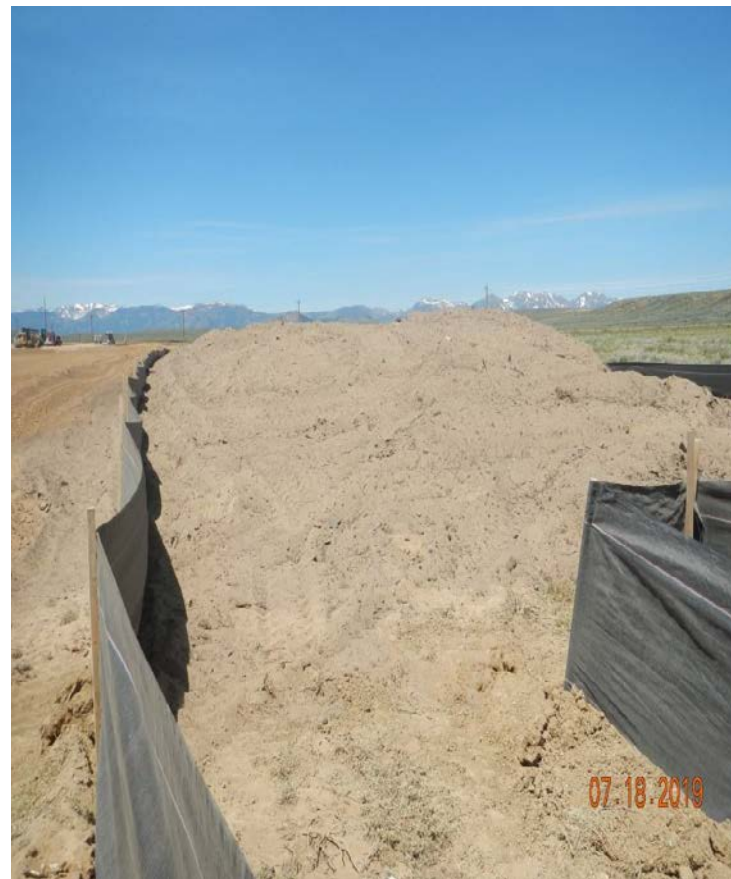
Photo#4: Silt fence; perimeter and topsoil stockpile BMP
