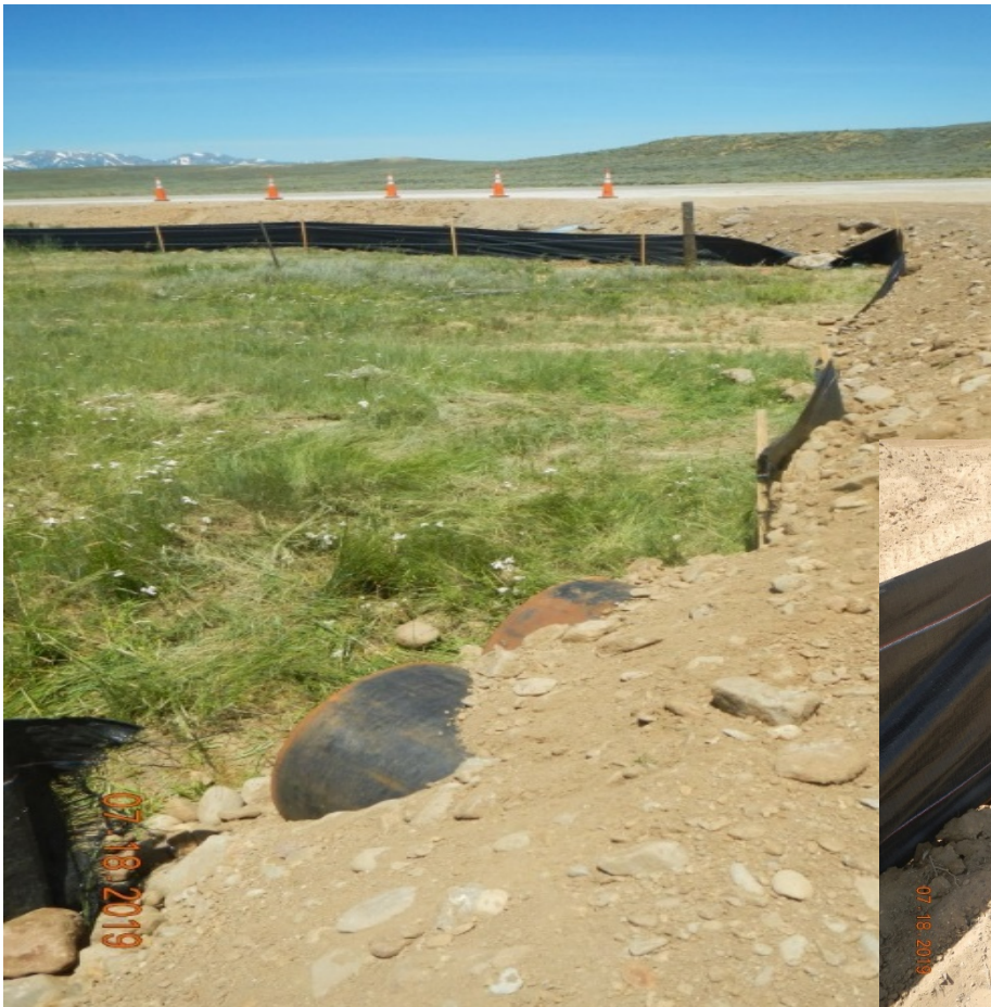
Photo#5: Culverts installed; sediment BMPs and silt fence repair needed.
