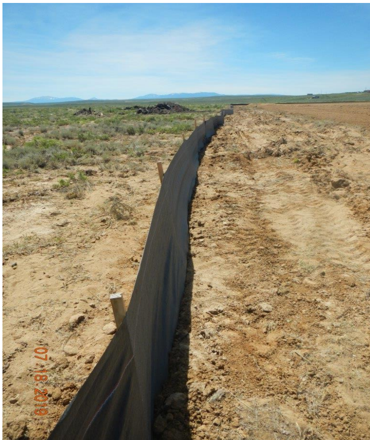
Photo#3: Silt fence; perimeter and topsoil stockpile BMP.
