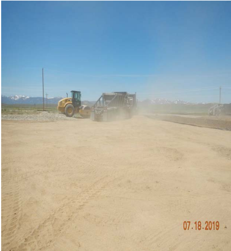
Photo#9: Fugitive Dust; water truck working.
