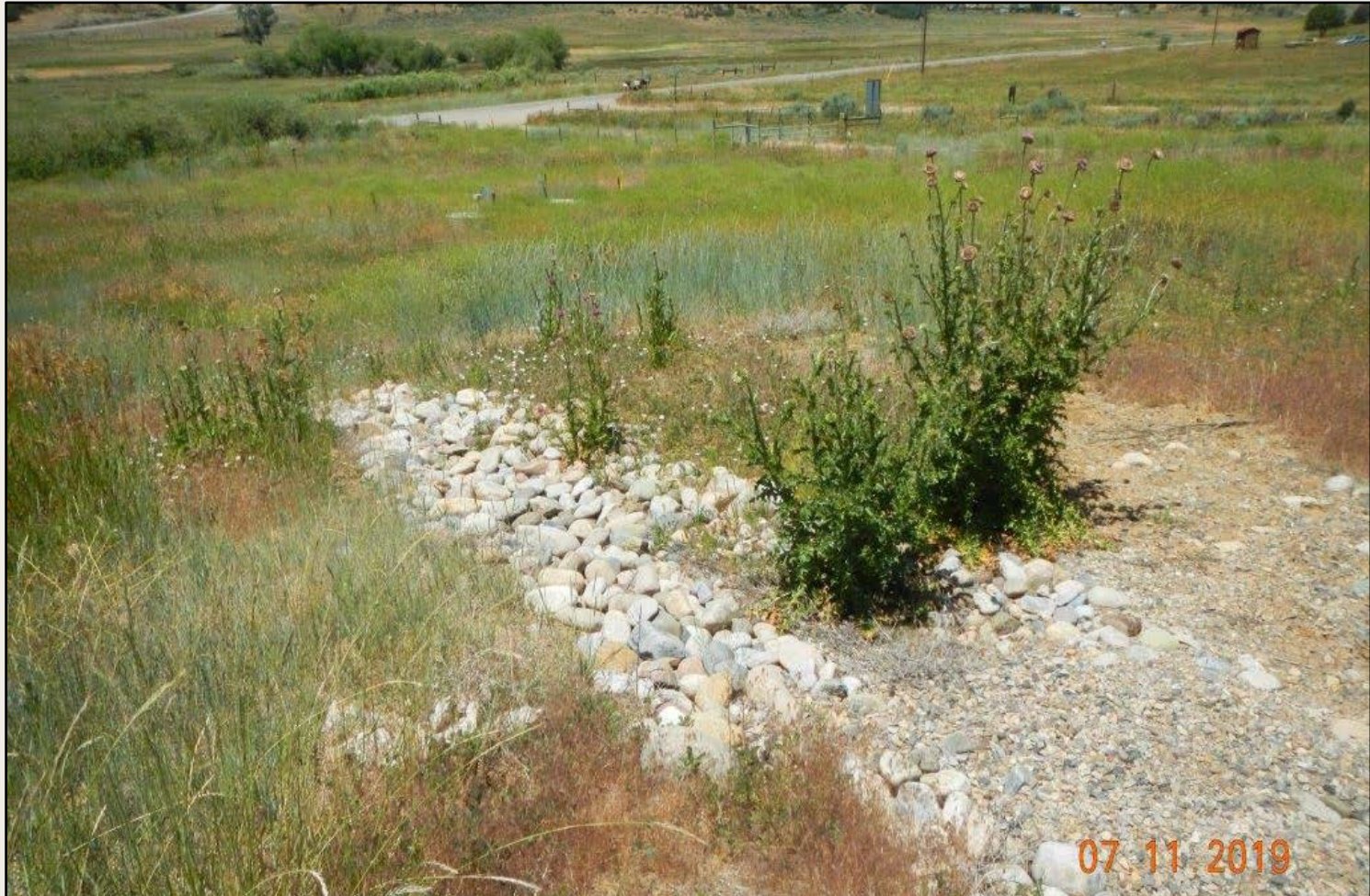
Photo 1. View of discharge point in the western project area. It appears gravel is being carried off of the well pad from high energy flows. This needs to be stabilized. Additionally approximately 200 musk thistles observed.
