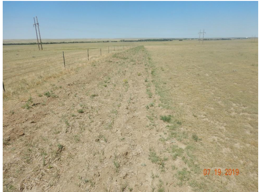
Photo 8: Photo taken from the access road. Photo shows reclamation in process.
