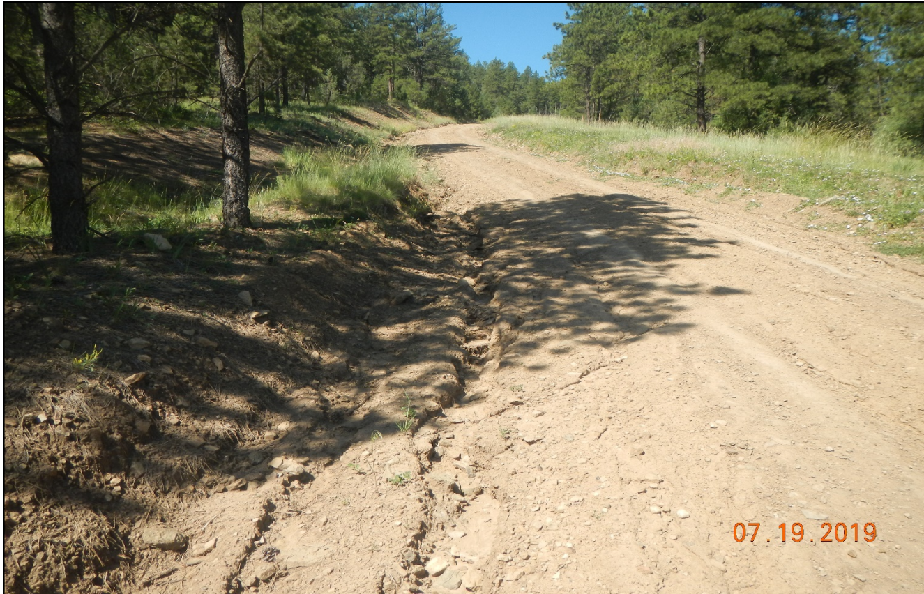
Photo 1. Stormwater is flowing down the road causing erosion. Corrective action was not performed since previous inspection.
