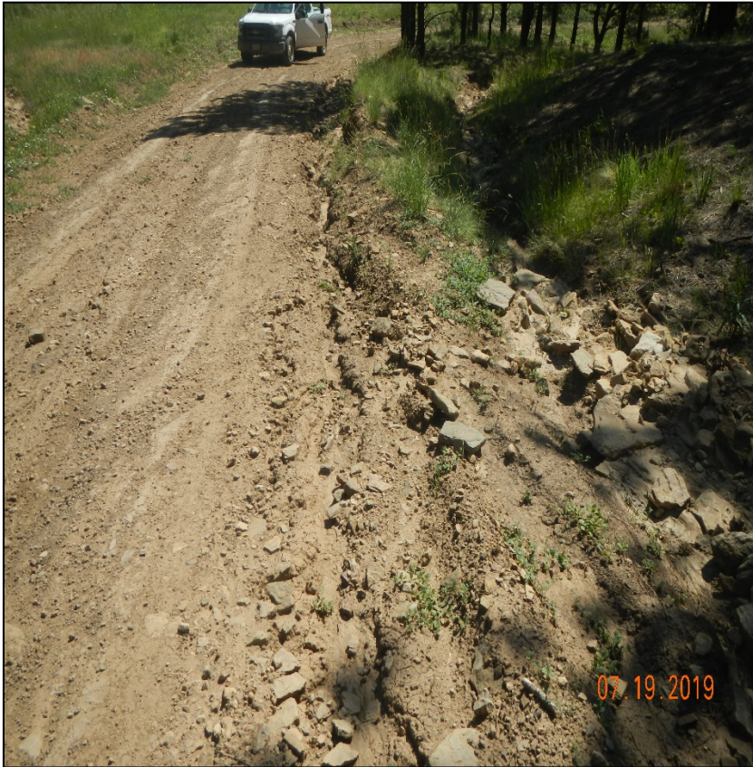
Photo 2. These two diversion ditches are transporting sediment offsite. No BMP's installed. Sediment trap or check damns would prevent sediment transport offsite. Corrective action was not performed since previous inspection.
