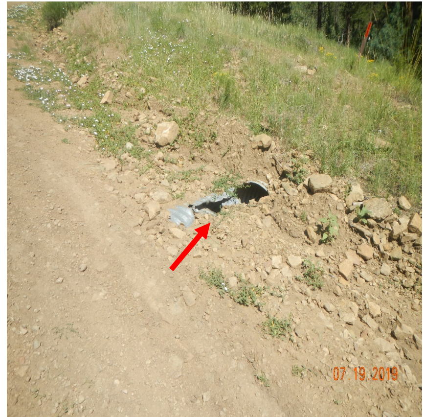
Photo 4. The photo on left is culvert inlet filled with sediment. Photo right is damaged culvert near outlet. Lat/Long:37.00845,-104.84245 Corrective action was not performed since previous inspection.
