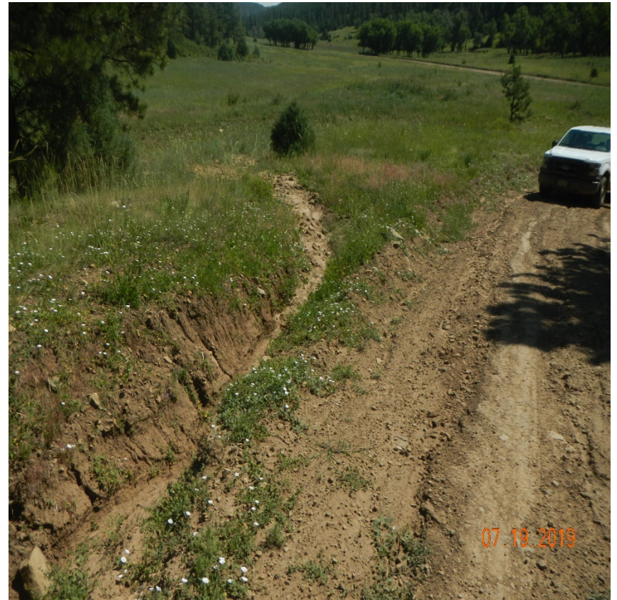
Photo 2. These two diversion ditches are transporting sediment offsite. No BMP's installed. Sediment trap or check damns would prevent sediment transport offsite. Corrective action was not performed since previous inspection.
