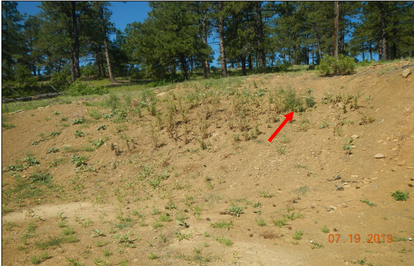
Photo 6. Facing toward the location. Red arrow points to List B noxious weeds. Some of the weeds were wilting from weed control but others were not treated. The cut slope is not stabilized.
