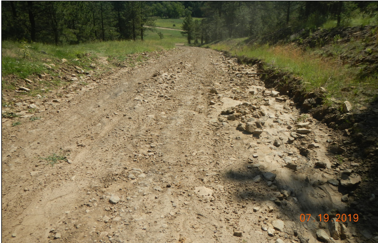
Photo 3. Stormwater is running down the road and is scouring the road. No BMP's installed. Corrective action was not performed since previous inspection.
