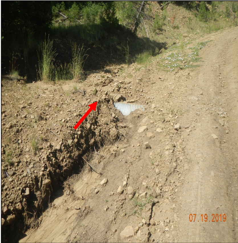
Photo 4. The photo on left is culvert inlet filled with sediment. Photo right is damaged culvert near outlet. Lat/Long:37.00845,-104.84245 Corrective action was not performed since previous inspection.
