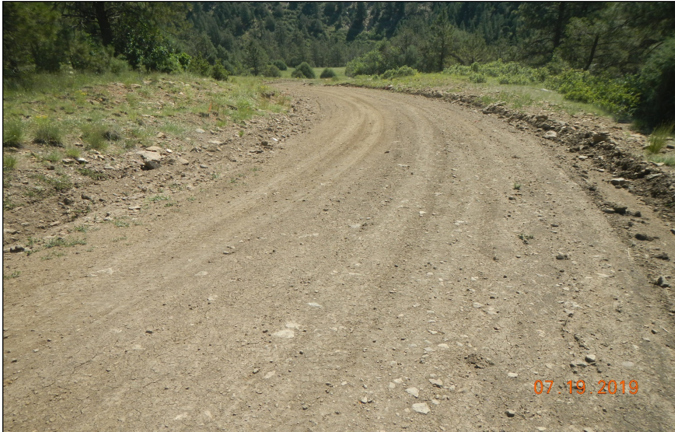
Photo 3. Road appears to have been graded but no BMP's are installed. Corrective action was not completed since previous inspection.
