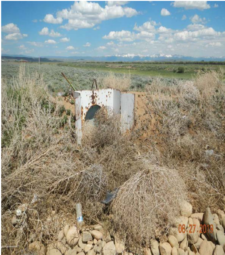
Photo#6: BMPs that are installed are ineffective.
