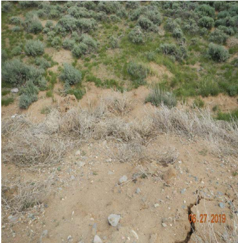
Photo#4: Sediment migrating off-site from base of berm.
