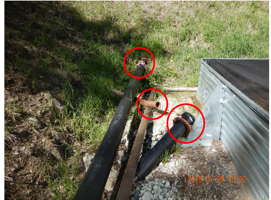
Photo #10 – Assorted flowlines located southwest of tank battery. Note unmarked HDPE and steel flowlines, two of which were uncapped on inspection date (circled in red).
