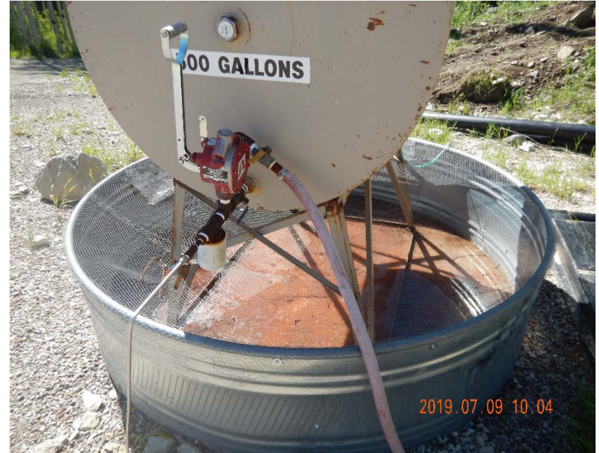
Photo #14 – 500 gallon methanol tank NE of tank battery inside of secondary containment. Note fluids inside of secondary containment device lacked hydrocarbon sheen and odor on inspection date.
