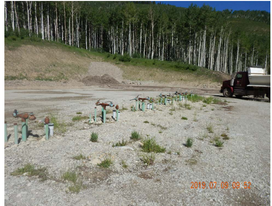
Photo #4 – Unmarked, unused flowline risers northwest of wellheads. Note uncontrolled vegetation growth in this area.
