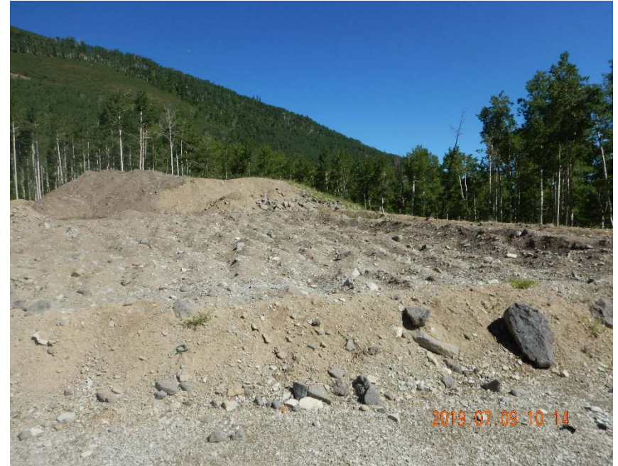
Photo #20 – Land treatment cell in northeast corner of pad.
