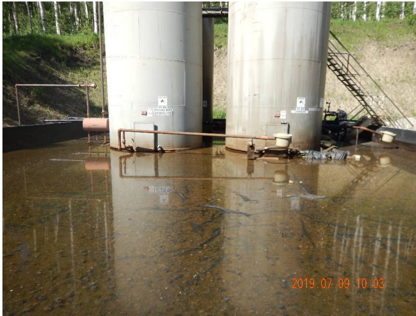
Photo #7 – Approximately 4” of fluids observed inside of tank battery containment area on inspection date. Hydrocarbon odors were noted in the area.
