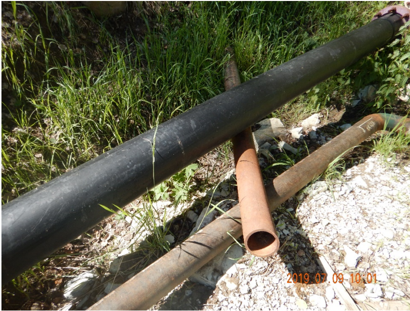
Photo #11 – Uncapped, unmarked 4” steel flowline from previous photo leads off-location to the south.
