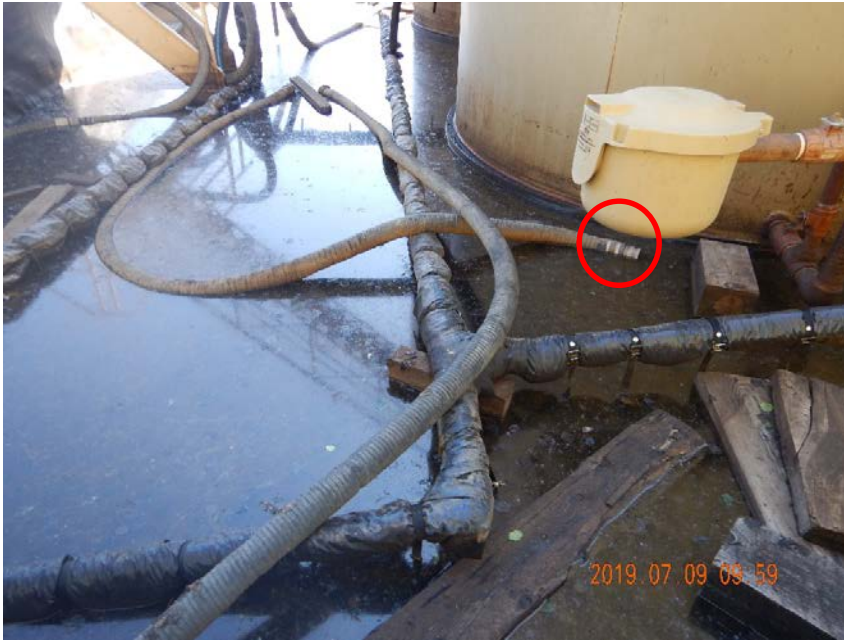
Photo #9 – Hoses and wood debris stored inside of tank battery secondary containment area. Note metal fittings on hoses.
