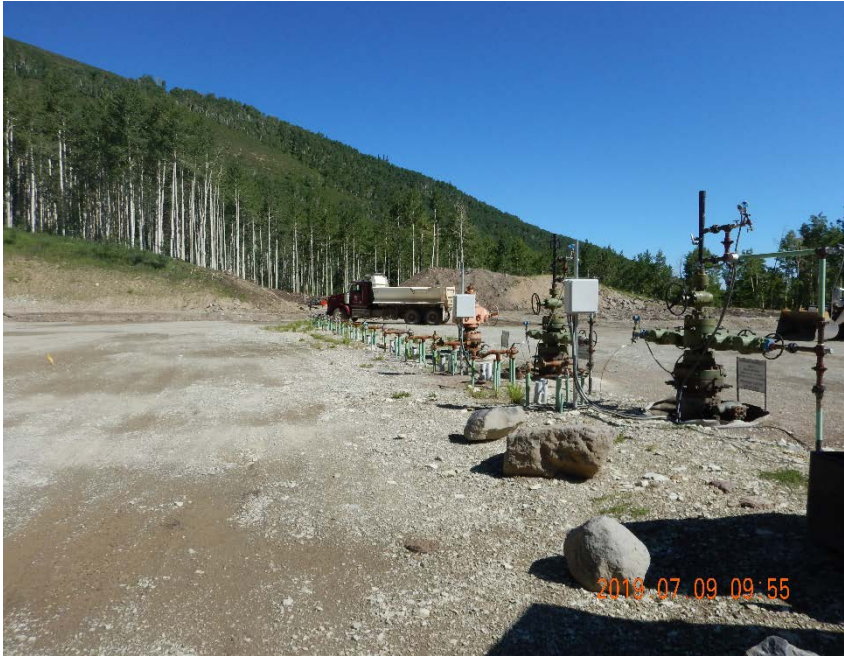
Photo #5 – Overview of wellheads and unmarked flowline risers in center of pad.
