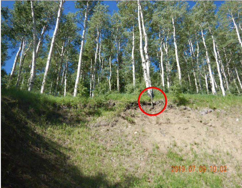
Photo #13 – View of aspen growth above cutslope in southwest corner of location (i.e., behind tank battery). Note exposed aspen root (red circle) and steep angle of cut slope.
