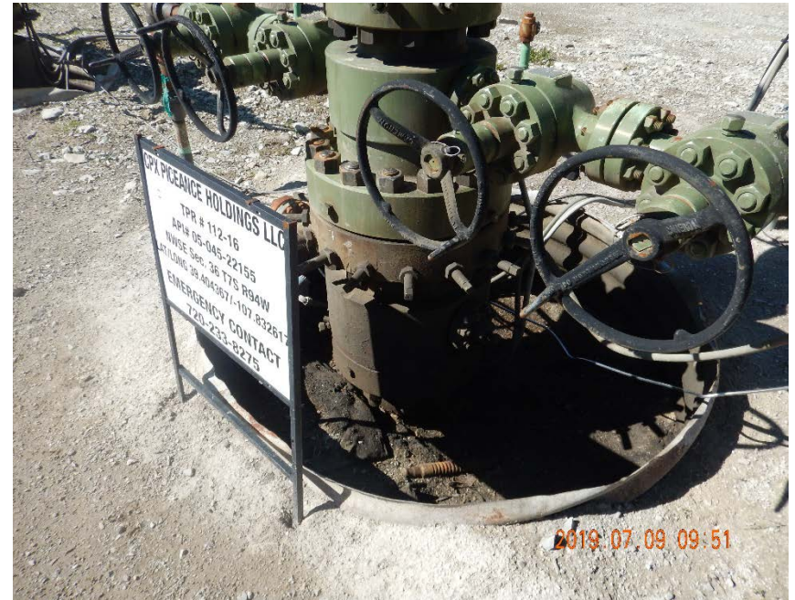
Photo #2 – TPR #112-16 wellhead, note open well cellar contains accumulations of oil-stained soil.
