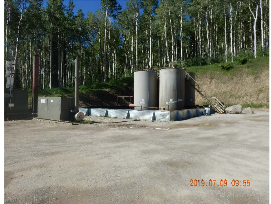
Photo #6 – Overview of tank battery and heated horizontal separators in southwest corner of location. Note vegetation growth beneath separator and along tank battery secondary containment device.
