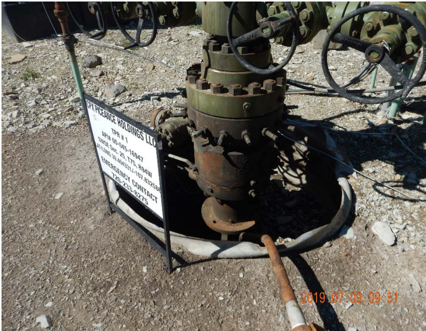
Photo #3 – TPR #1 wellhead. Accumulations of oil-stained soil observed inside open well cellar on inspection date.
