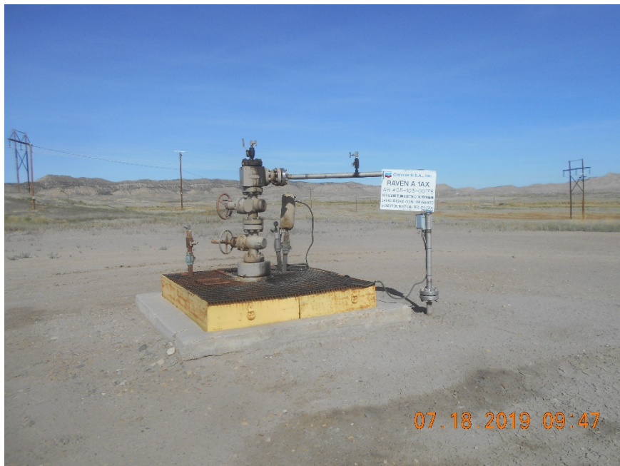
Injection wellhead
