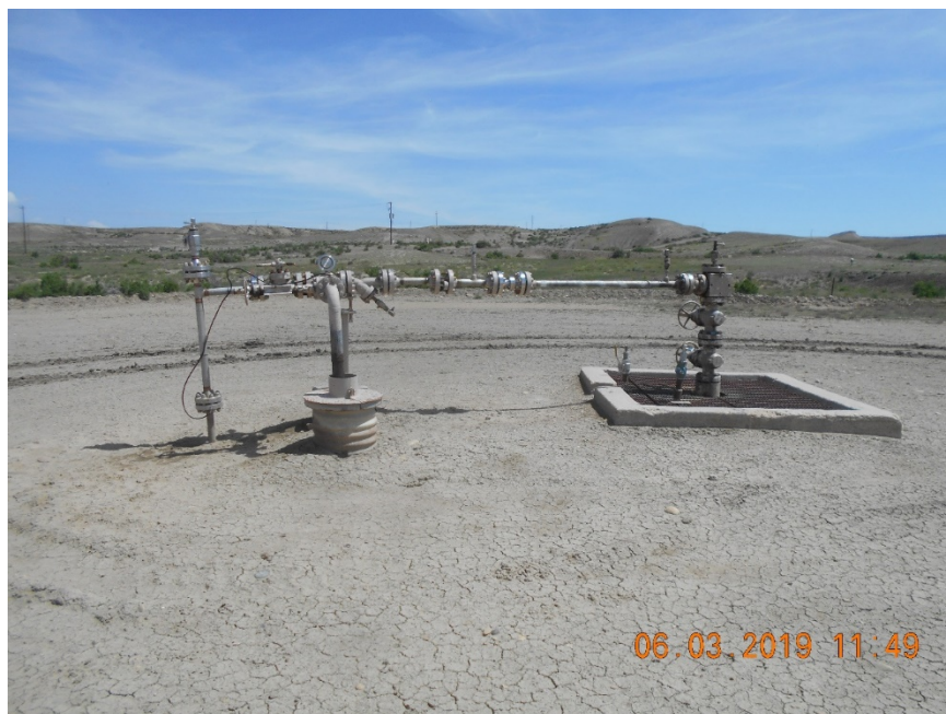
Injection wellhead - Missing sign. Inspection photo 6/3/2019
