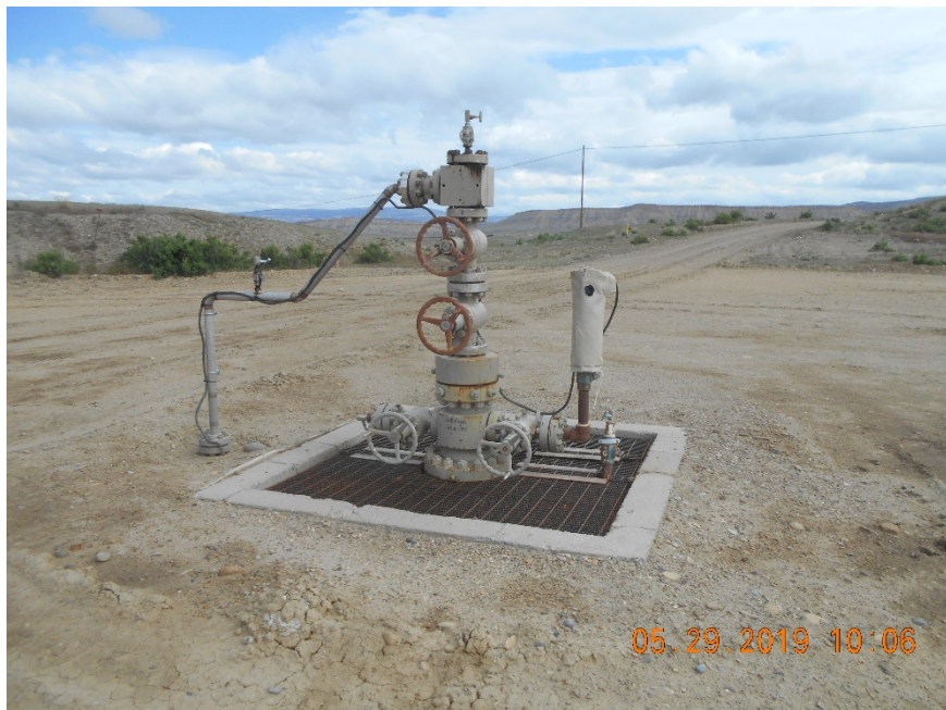
Injection wellhead – Missing sign. Inspection photo 5/29/2019
