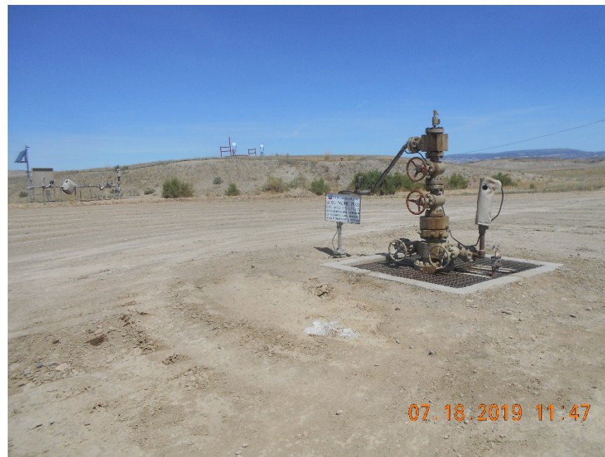
Injection wellhead – CA completed. Inspection photo 7/18/2019
