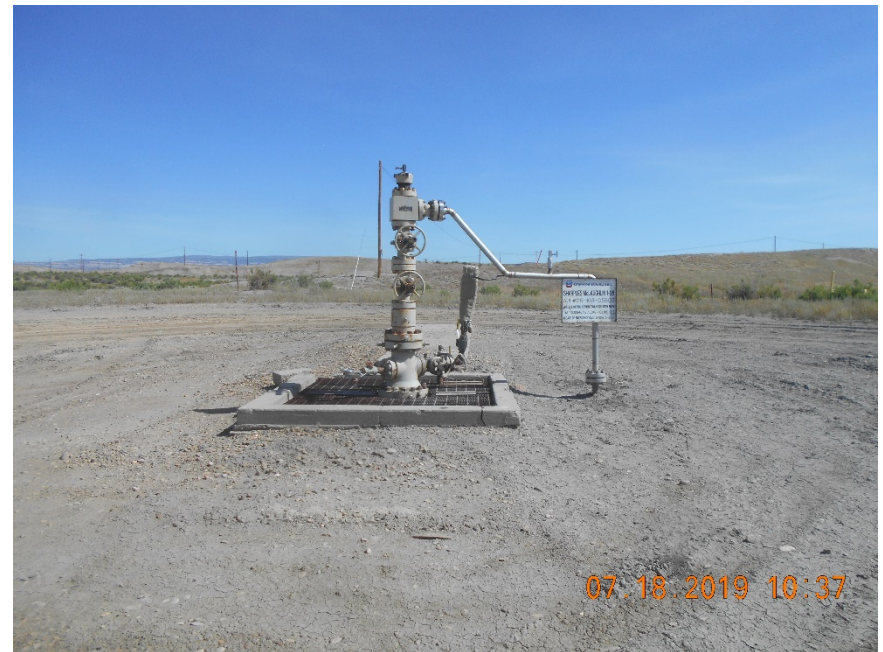
Injection wellhead. CA completed. Inspection photo 7/18/2019
