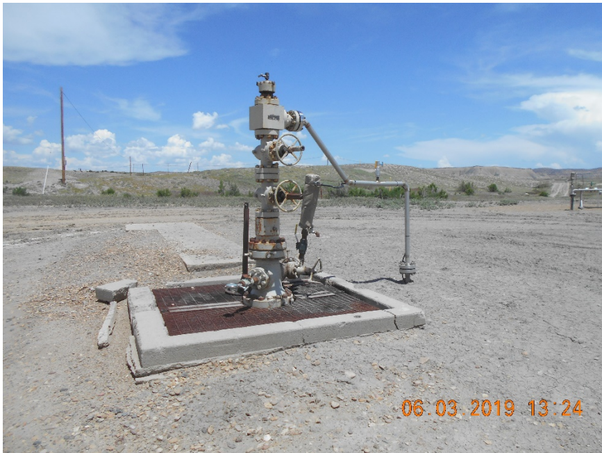
Injection wellhead - Missing sign. Inspection photo 6/3/2019
