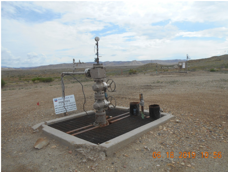
Injection wellhead. Trash buckets on cellar grate. Inspection photo 6/18/2019
