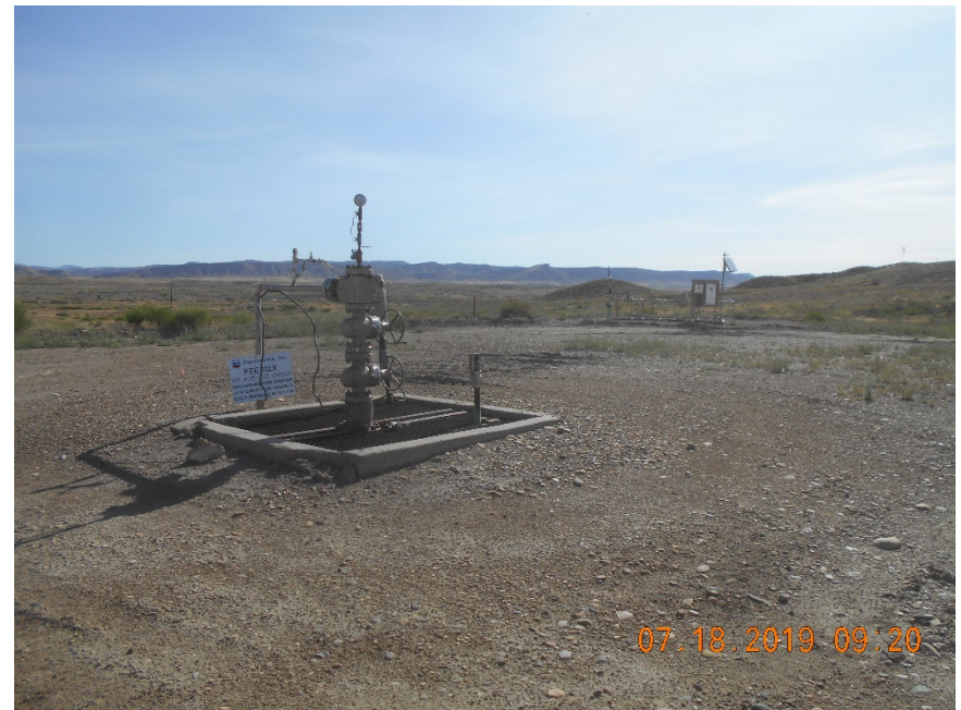
Injection wellhead. Trash removed. CA completed Inspection photo 7/18/2019
