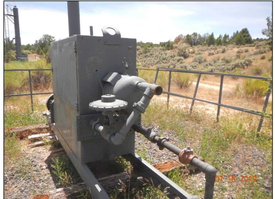
**Photo # 6 Separator out of service , part on the ground at time of inspection.**
