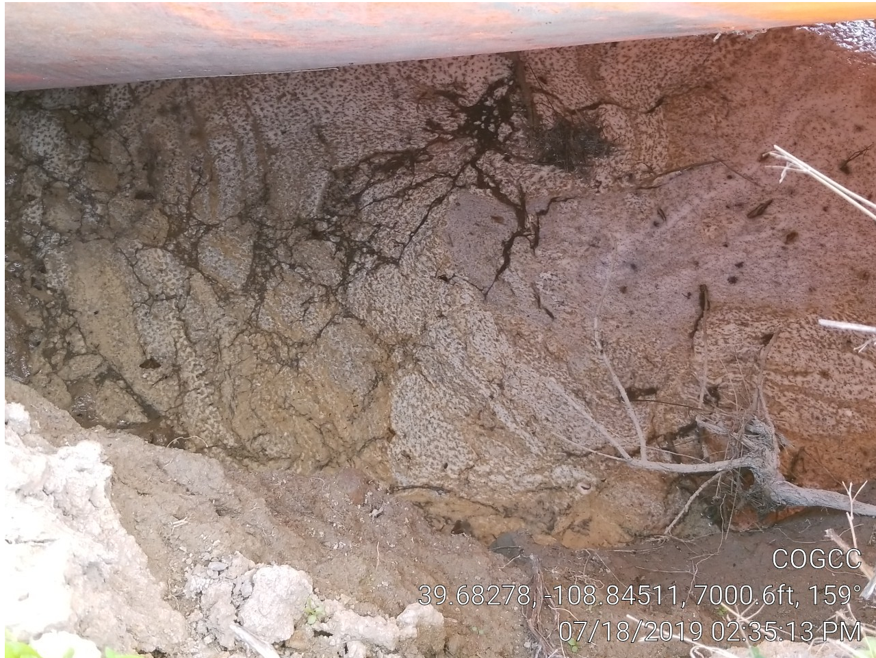
Photo 2. Fluid in hole where the blowdown was occupying the space.
