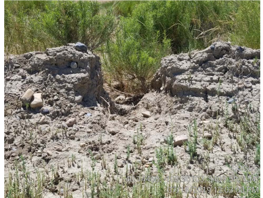
Photo 3. Break on location berm.
