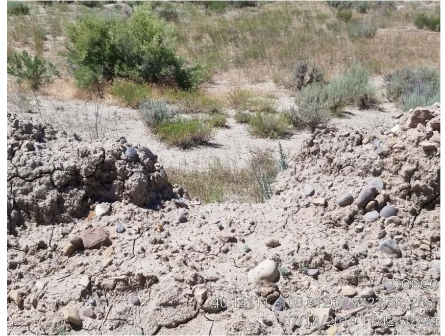
Photo 3. Break in location berm.
