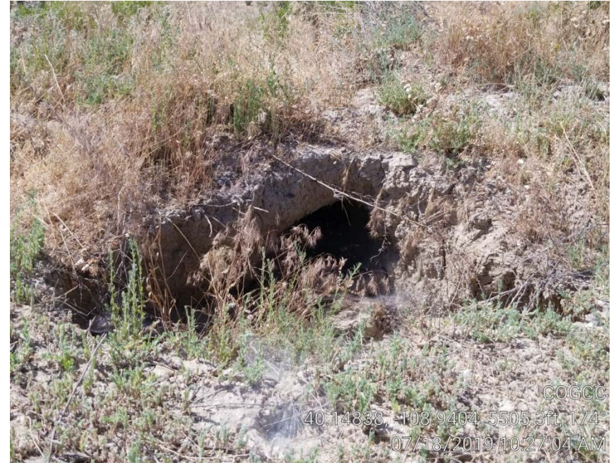
Photo 3. Hole in location berm.
