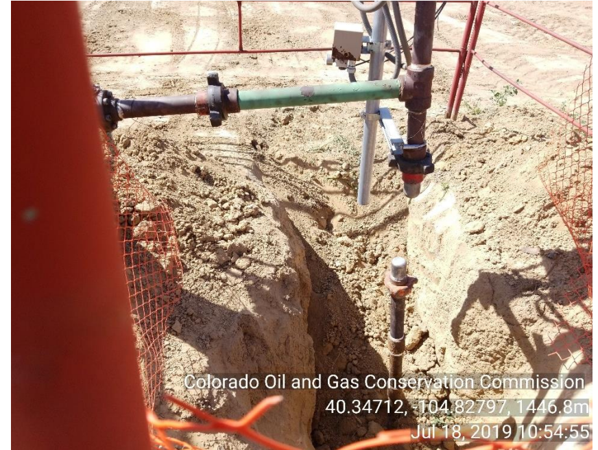
Photo 2 At time of inspection crew was on site performing repair on flow line.
