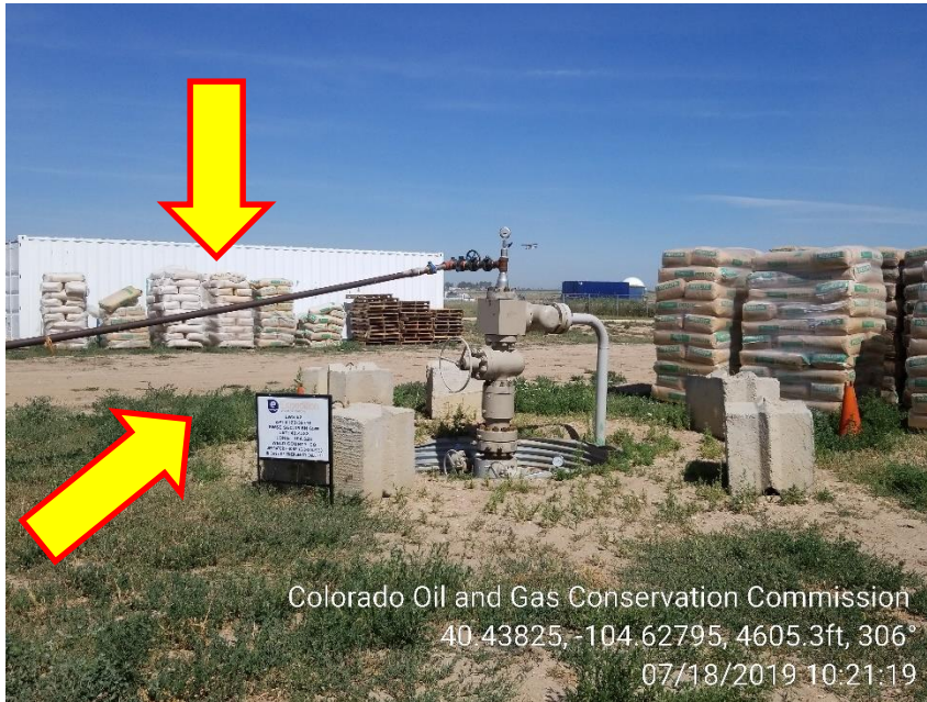
Photo 1 – Weeds at Wellhead, Perlite not in Containment
