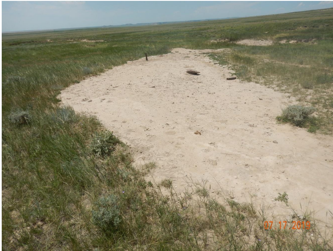
Photo 2: Photo taken from the well location, facing west. Photo shows riser remaining at location. Photo also shows location remains bare and exposed soil. Unable to find evidence that reclamation has been conducted per corrective actions.
