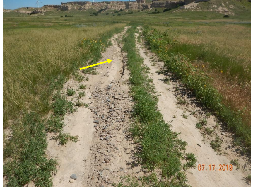
Photo 6: Photo taken from the access road, facing northwest. Photo shows stormwater erosion degradation evident. Photo also shows reclamation activities, including but not limited to, compaction alleviation, recontouring/regrading and revegetation activities have not been conducted.
