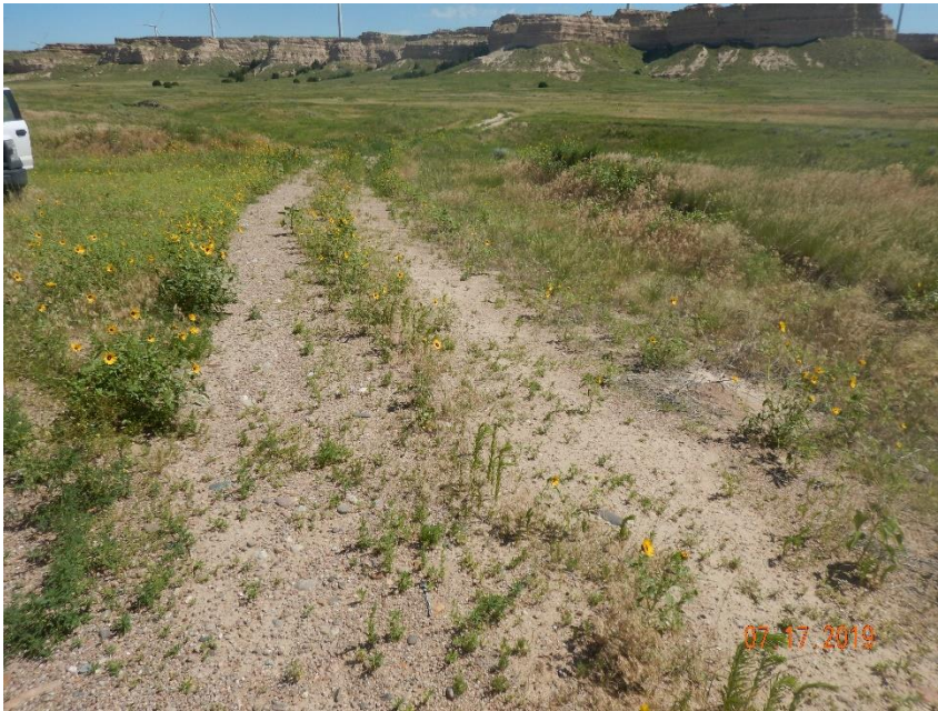
Photo 7: Photo taken from the where the well access road intersects with the main access road. Photo shows access road has not been reclaimed.
