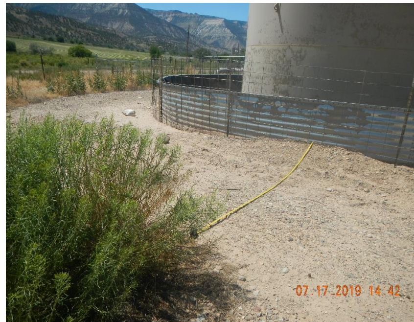
Weeds growing within less than 25 ft of tanks.
