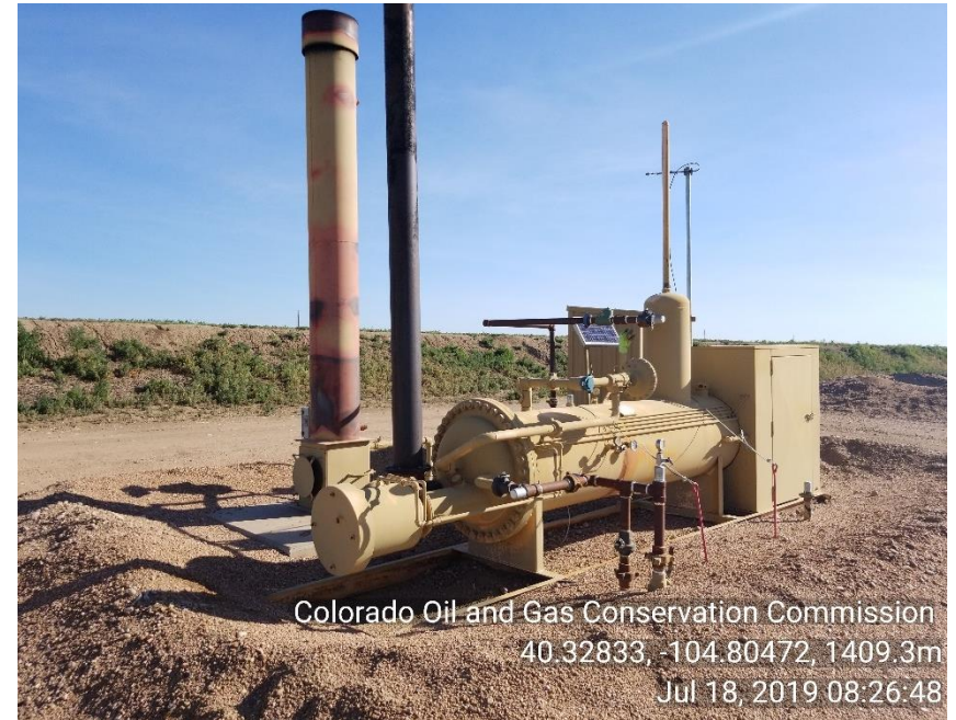
Photo 2 Sep/meter house and ECD
