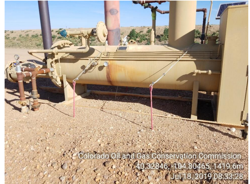
Photo 6 HOZ Sep anchoring installed
