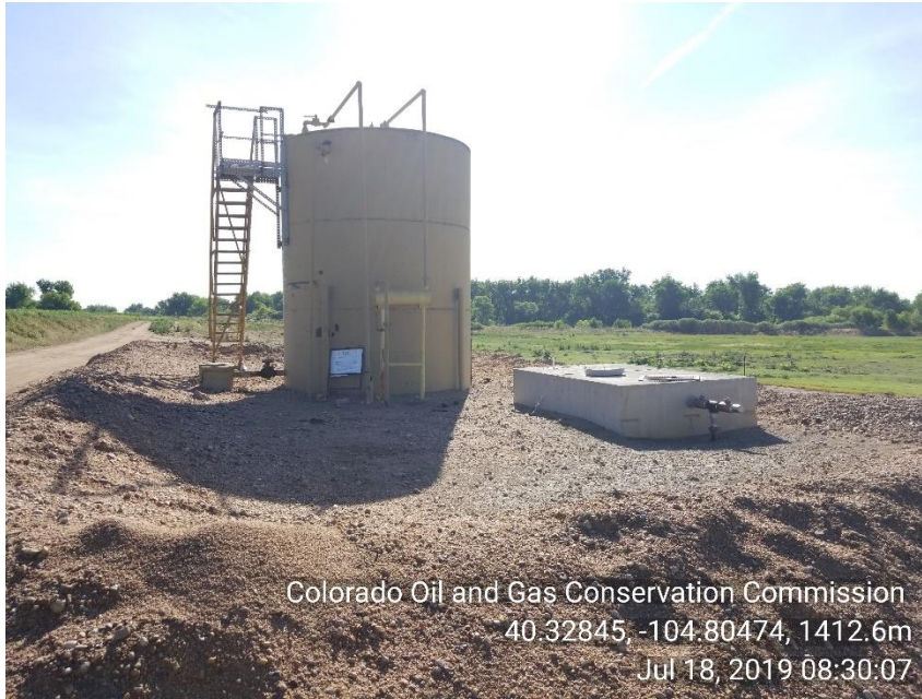
Photo 3 TNK BTRY located in floodplain does not have steel containment.
