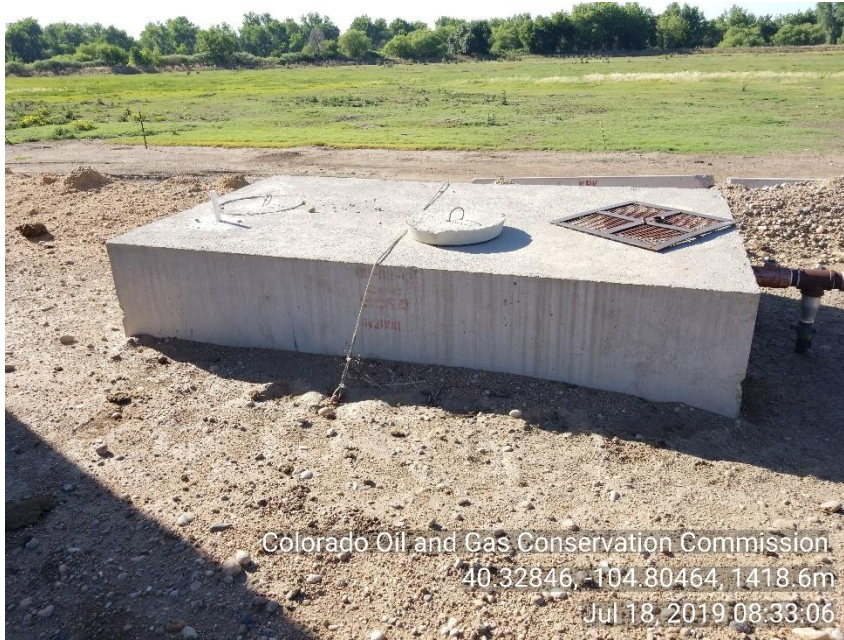
Photo 5 Produced water tank Anchoring installed.
