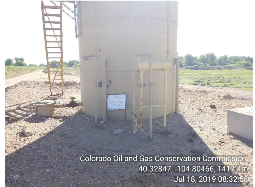
Photo 4 TNK BTRY in floodplain and does not have proper anchoring.
