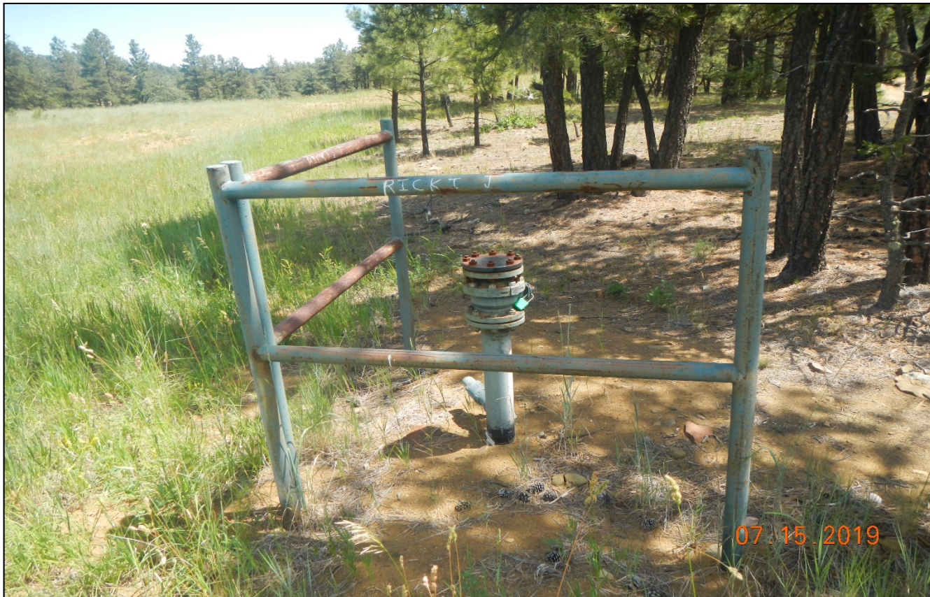
Photo 2. Pipe riser remains near the location. Pipe riser needs to be removed per the condition of approval.
