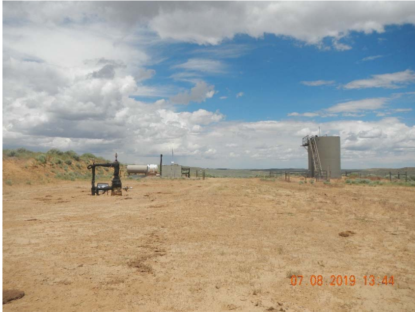
Photo 3. Overview of location taken from south side facing north.
