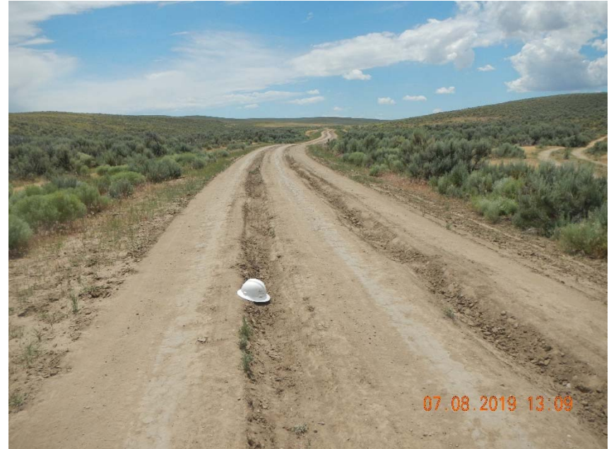
Photo 4. Ruts in access road, hard hat for scale.
