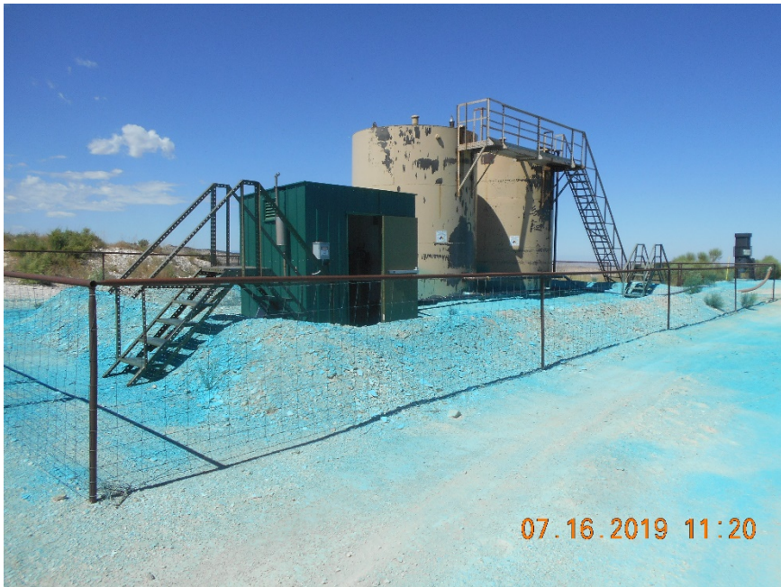
Pump housing and Tank battery
