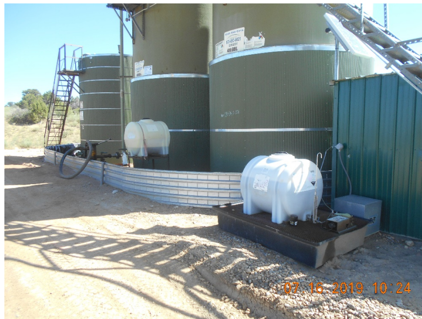
Tank battery and Secondary containment of chemicals
