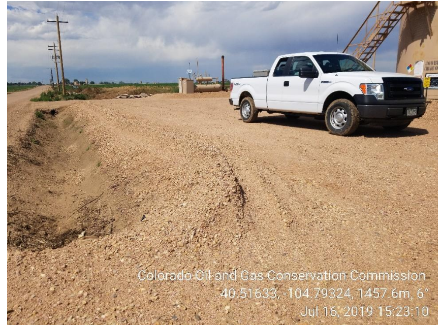
Photo 4: Erosion is repaired
