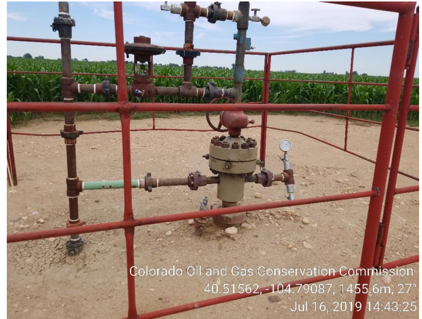
Photo 2: Unused equipment removed
