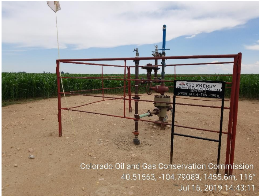
Photo 1: Wellhead; unused equipment removed
